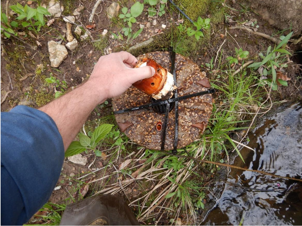
Photo 6. PVC pipe being removed from the bottom of the concrete housing (April 14, 2021).
