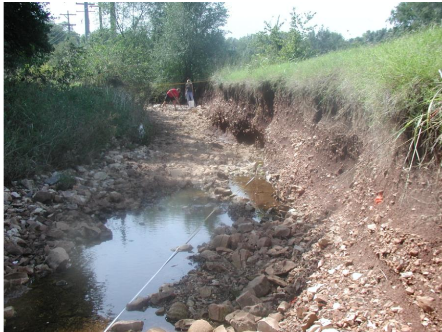
Photo 2. Bank erosion monitoring through golf course reach
