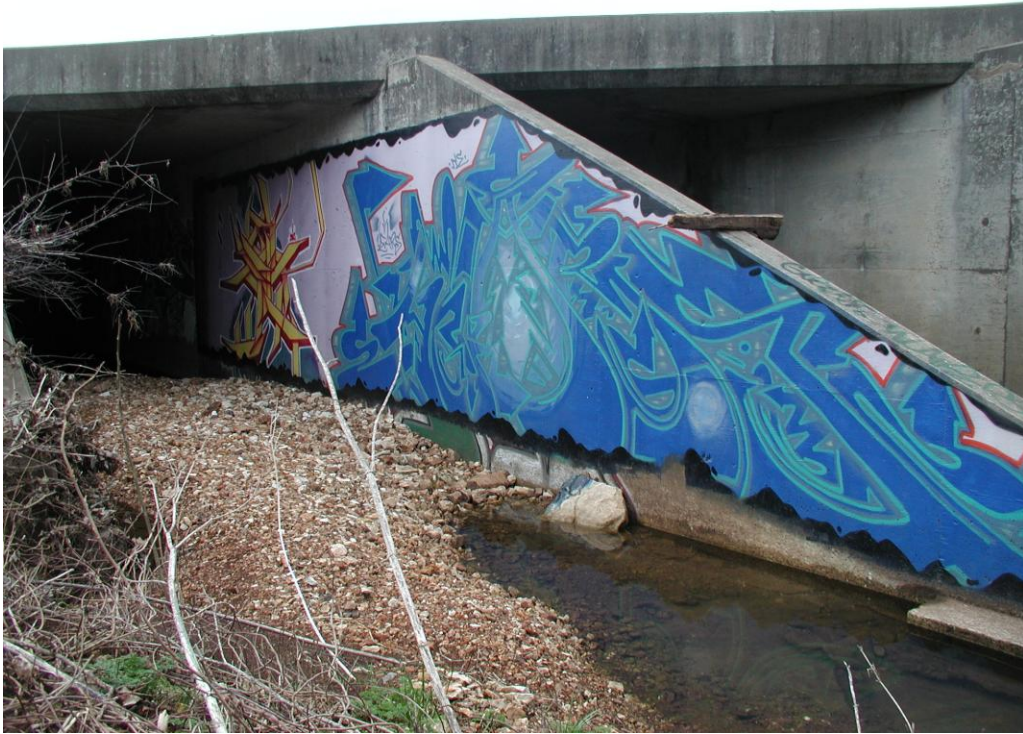
Photo 5. Site 5 upstream of bridge at Campbell
