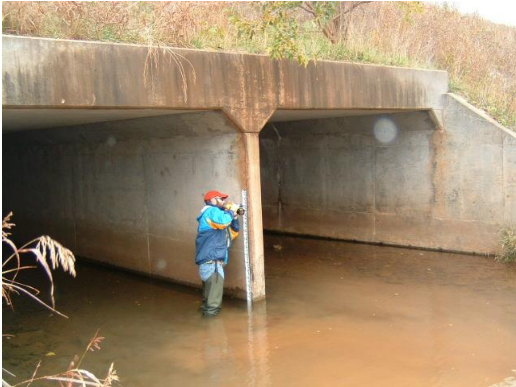
Photo 1. Site 1 below the Republic Road culvert
