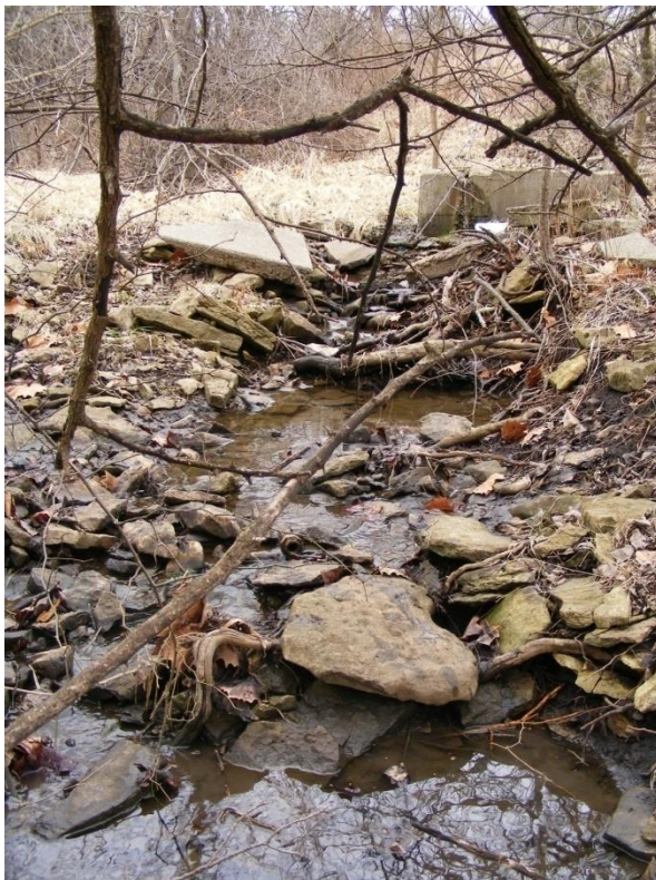
Photo 6. SR-4a looking downstream at headcut near concrete stock tank (Feb. 2008)
