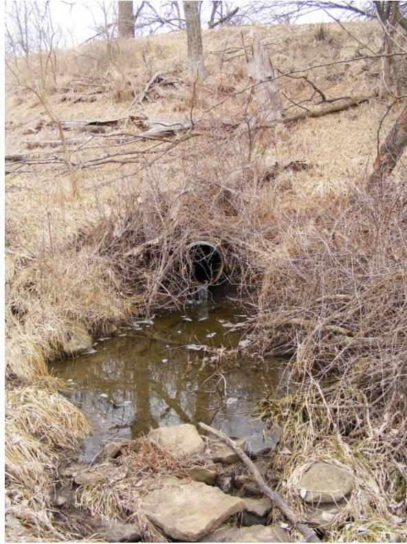
Photo 1. Pond dam outlet begins SR-1 (Feb. 2008)
