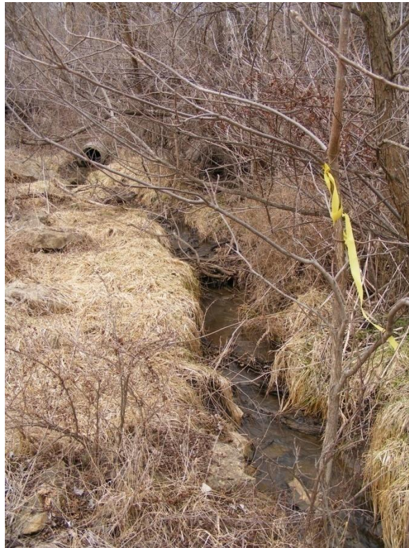
Photo 16. SR-8 begins below rubble dam outlet (Feb. 2008)
