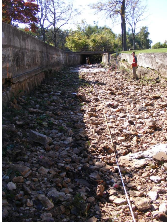
Photo 3. Looking downstream at SR-3 near station 1,100 feet (10/16/2008)
