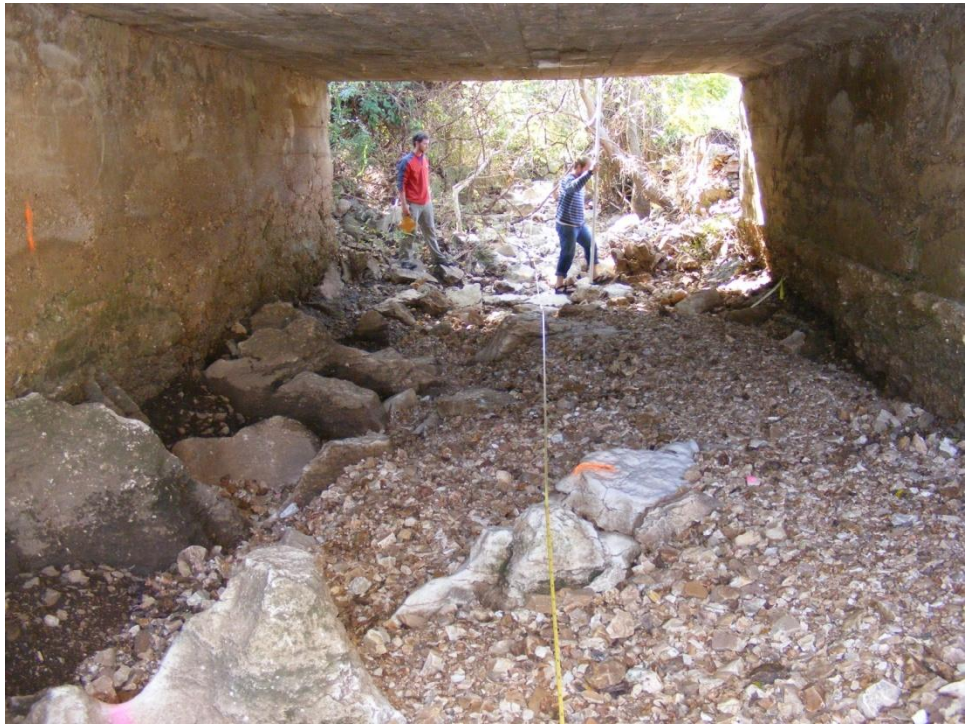
Photo 6. Looking downstream at SR-2 near station 900 feet (10/16/2008)
