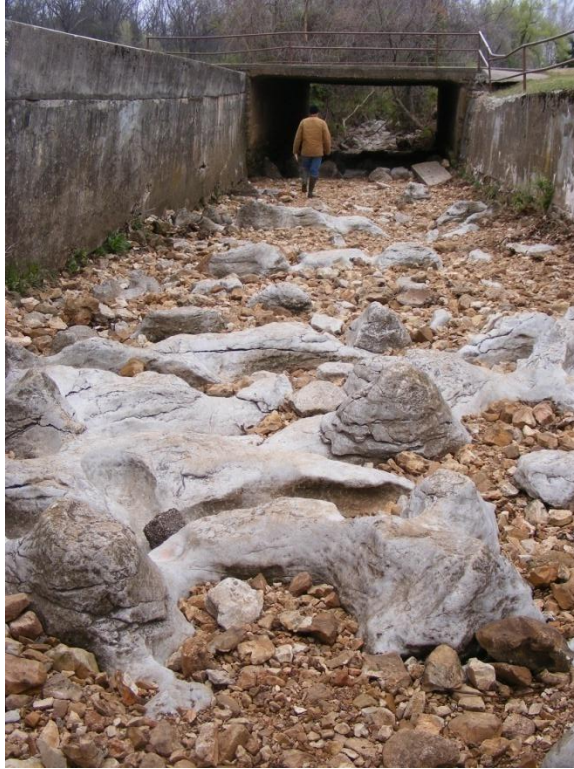
Photo 28. Bedrock pinnacles near station 900 feet looking downstream SR-2 (4/6/09)
