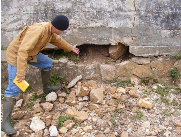
Photo 24. Cobble and coarse gravel source from backfill of failing wall along left bank near SR-3 station 1,200 feet (4/6/09)
