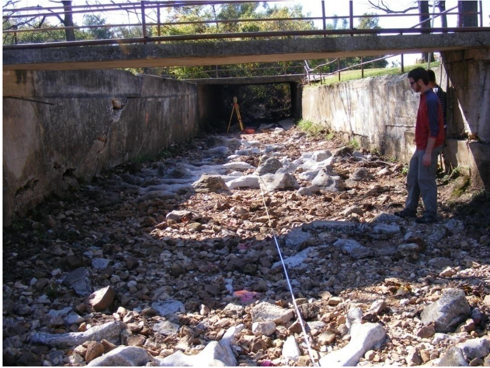
Photo 5. Looking downstream at SR-2 near station 1,000 feet (10/16/2008)
