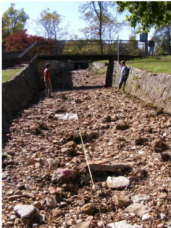
Photo 2. Looking downstream at SR-3 near station 1,200 feet (10/16/2008)
