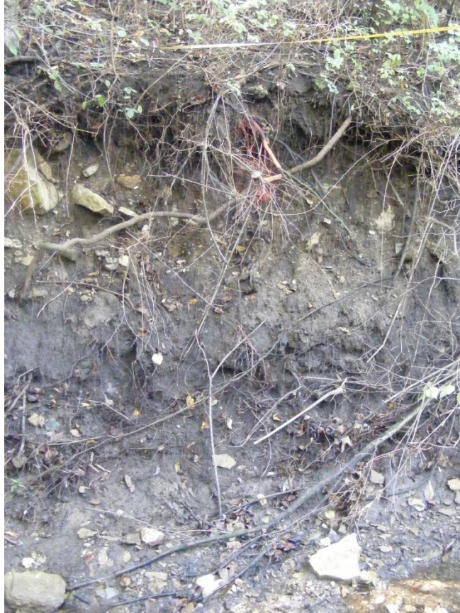
Photo 27. R11 - xs 11, St. 3,710 ft right bank (Sept. 2009)
