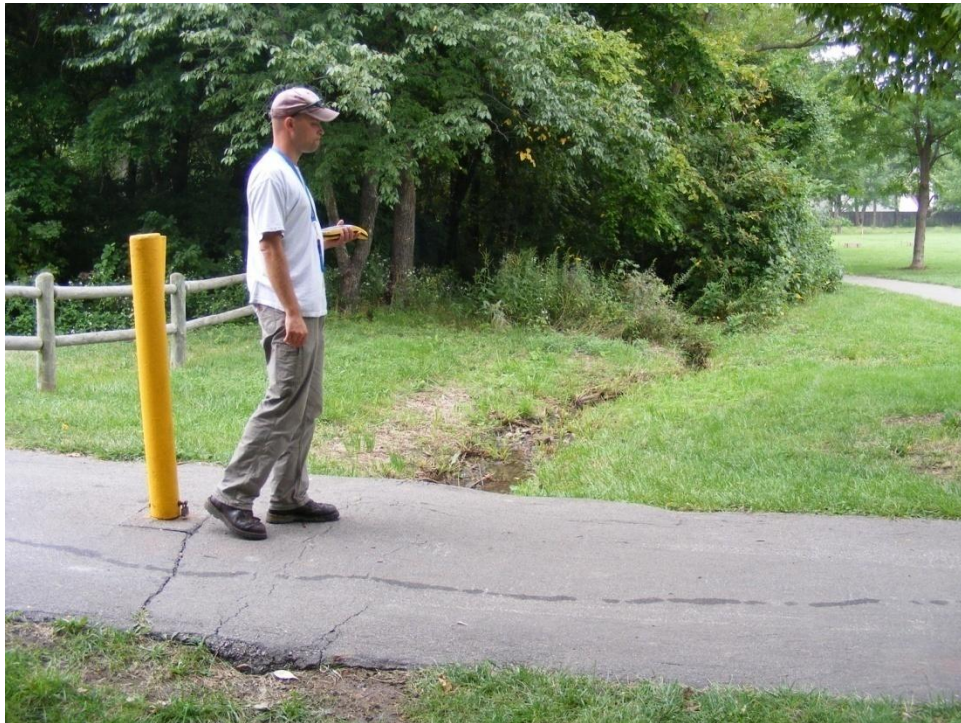
Photo 2. R1-A Path at St. 7,550 looking downstream (Sept. 2009)
