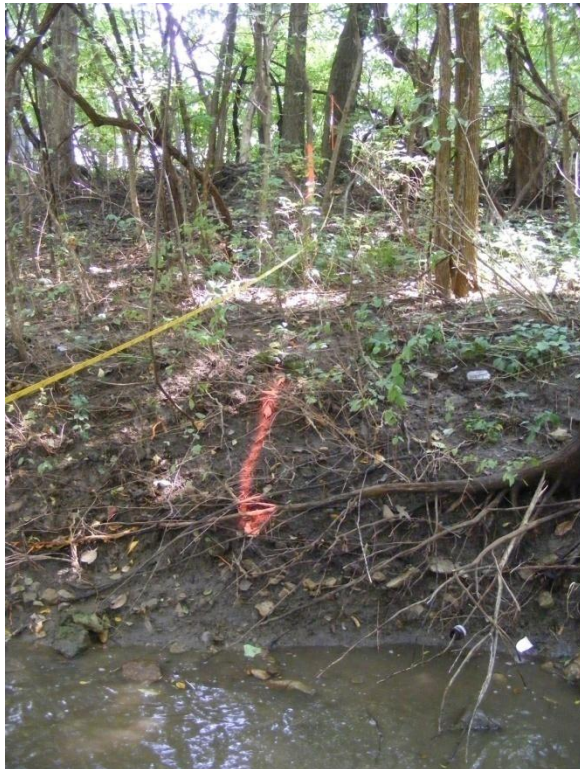
Photo 40. R14 – xs 14 St. 2,140 ft right bank (Sept. 2009)
