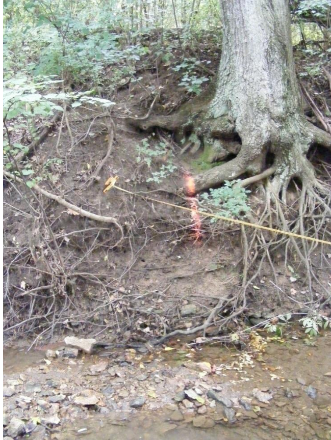
Photo 53. R15-B xs 17 St. 320 ft right bank (Sept. 2009)
