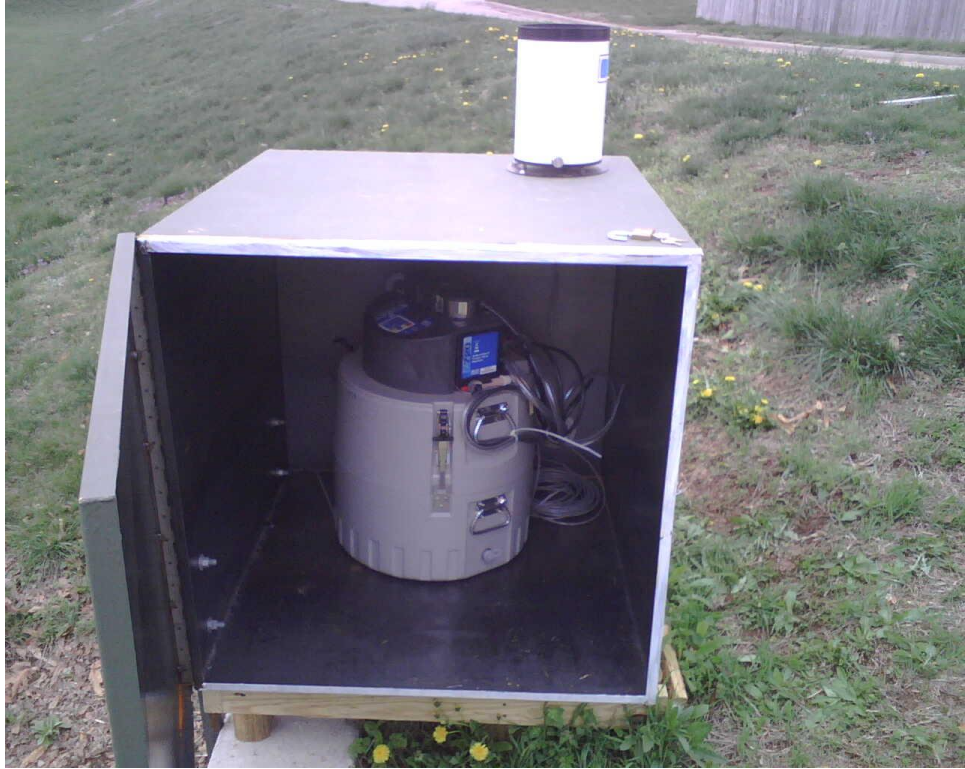
Photo 5. Installation at Park Hill Subdivision in Nixa
