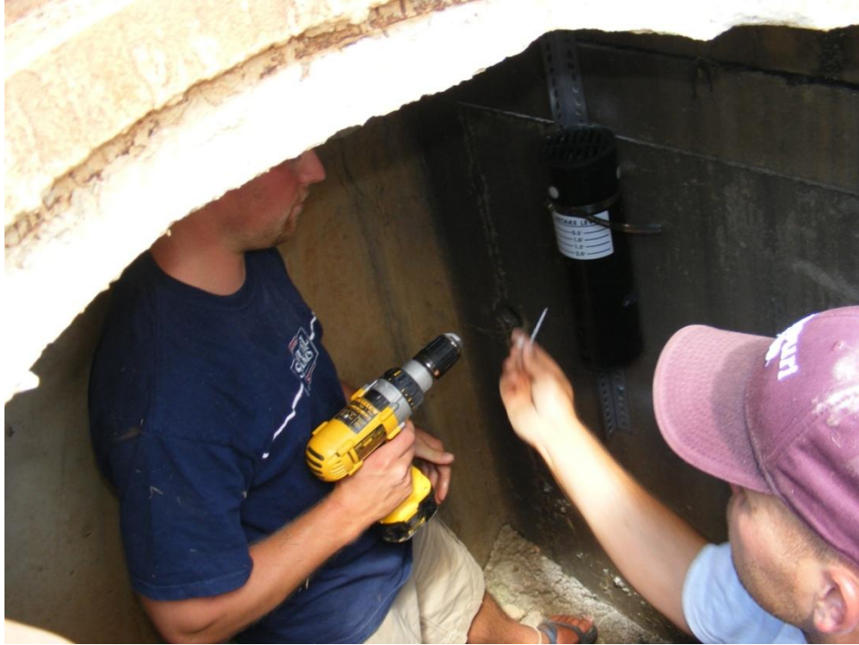
Photo 9. Installation of curb inlet sampler at Park Hill
