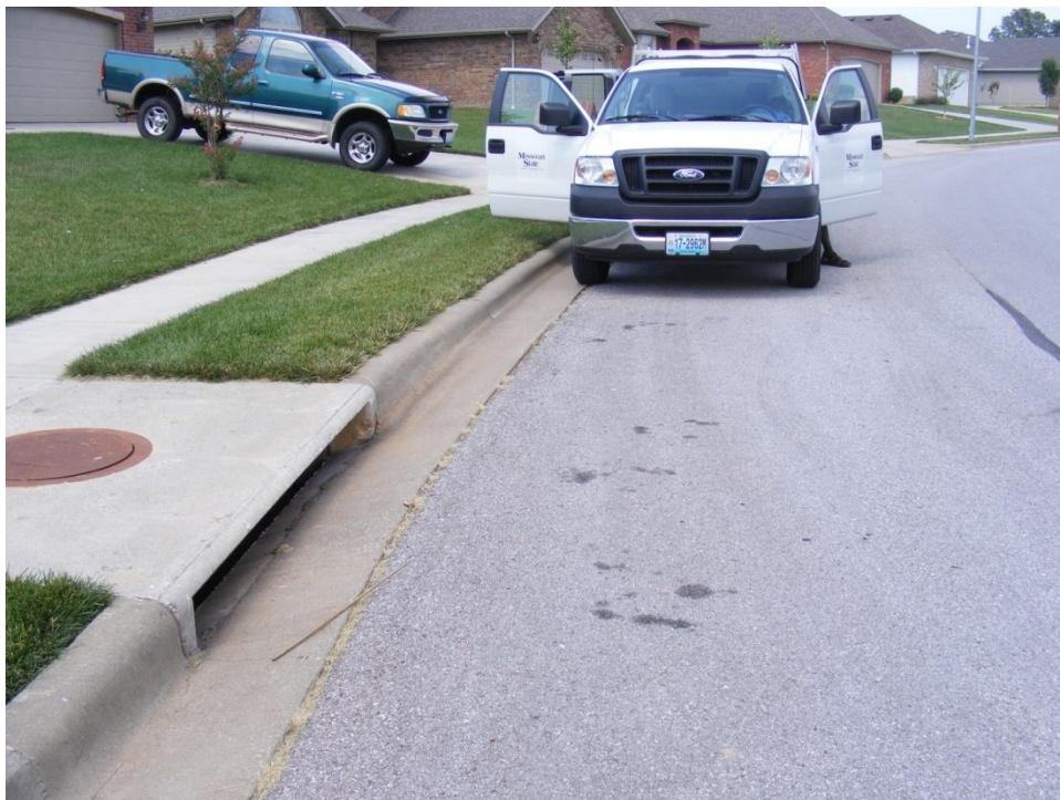
Photo 8. Inlet where curb samplers were installed
