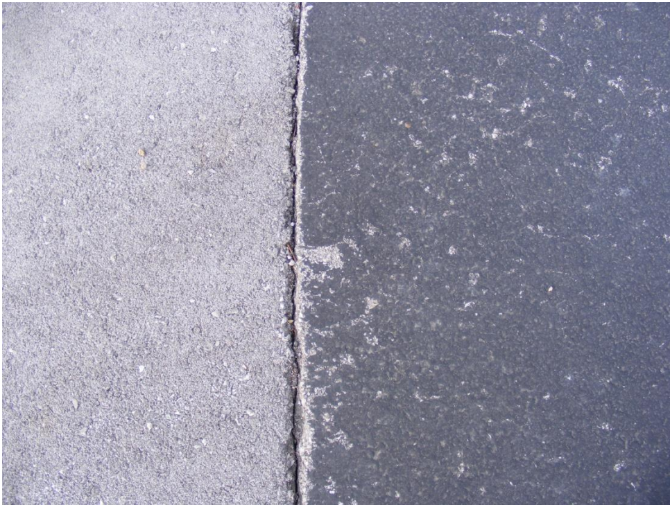
Mixed Asphalt(unsealed) and Seal-coated Lot
