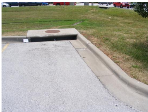
Parking lot above sample 49
