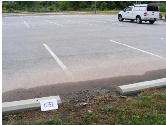
Parking Lot above sample 31
