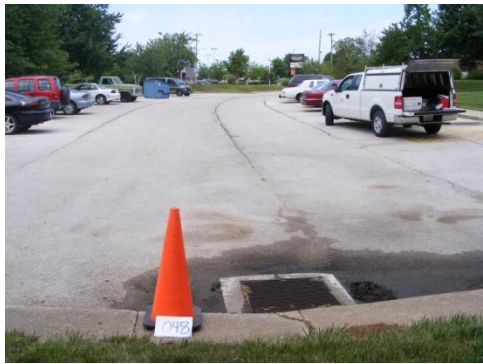
Parking lot above sample 48
