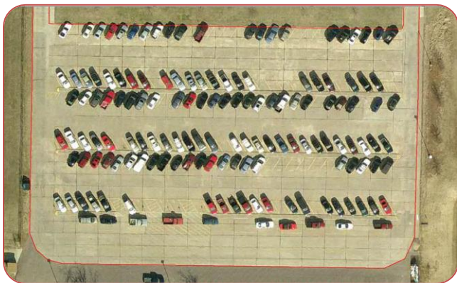
Concrete Lot (unsealed) on 2009 Aerial Photograph
