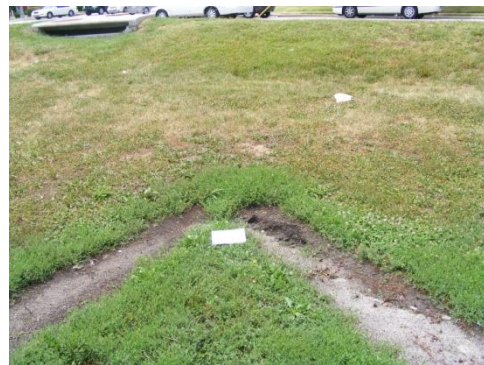
Sample 49- basin channel bed
