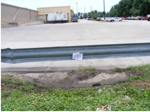
Parking lot above sample 50
