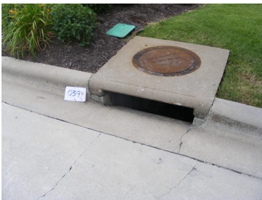
Parking lot outfall above sample 39
