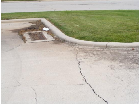
Parking lot above sample 47
