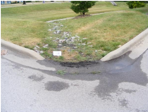
Parking lot and outfall near sample 38
