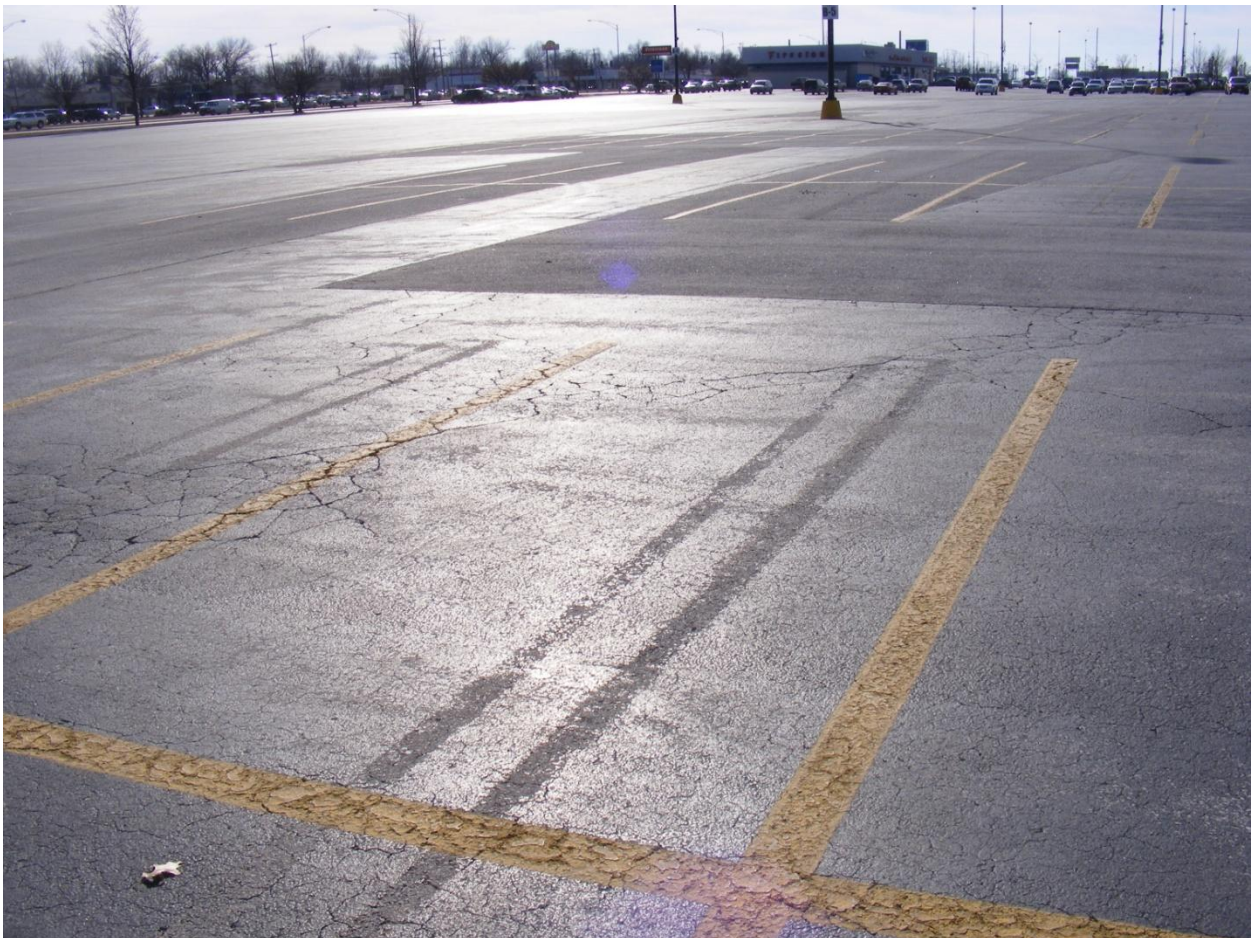
Mixed sealed and asphalt parking lot
