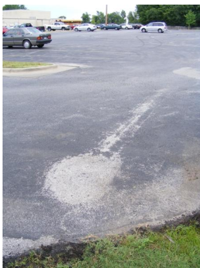
Parking lot above sample 41
