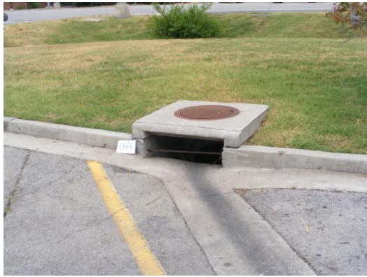
Parking lot outfall above sample 44
