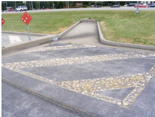
Parking lot outfall above sample 45
