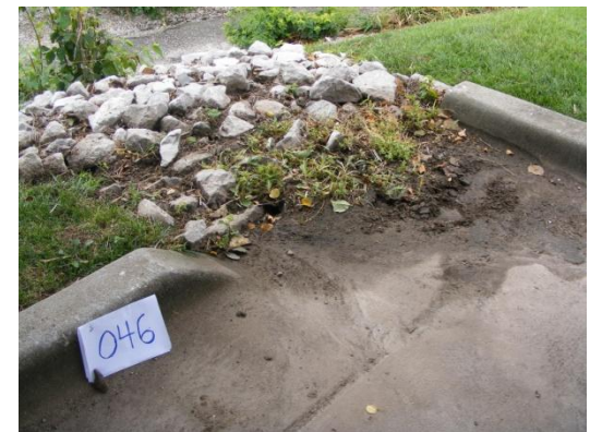
Sample 46- lot edge at outfall
