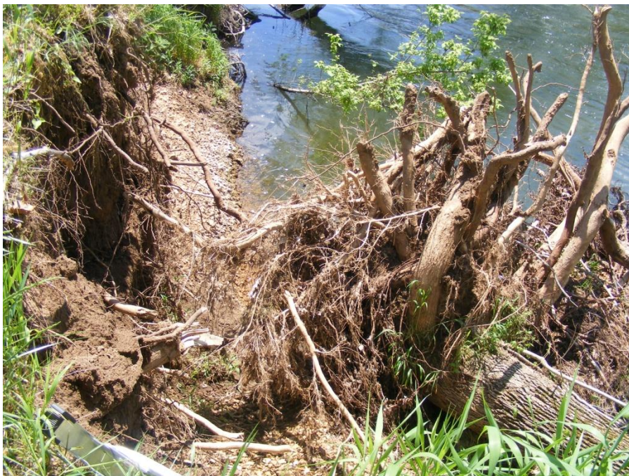
Photo 10. Recently downed tree after bank failure, May 2013.
