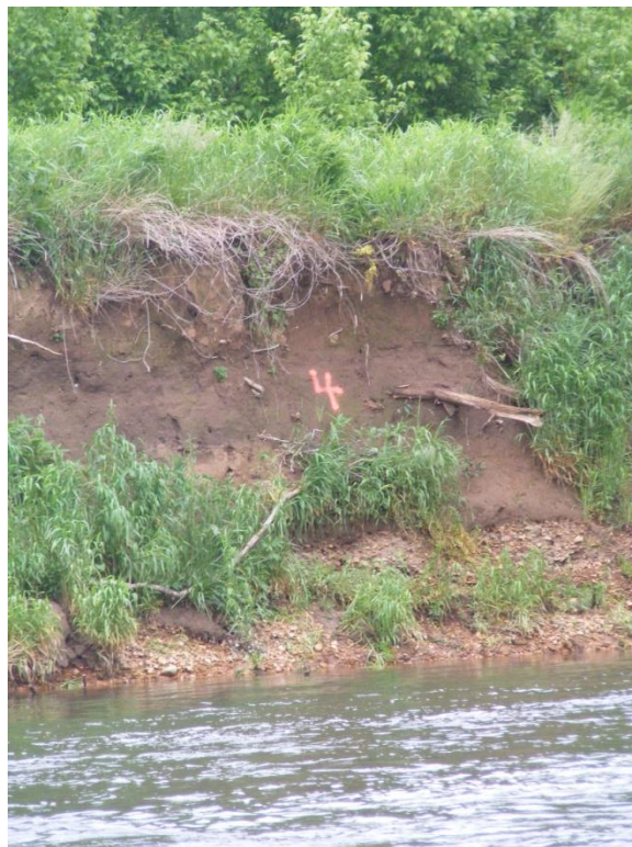
Photo 8. Erosion pin transect 4 at high flow, willows under water, May 2013.
