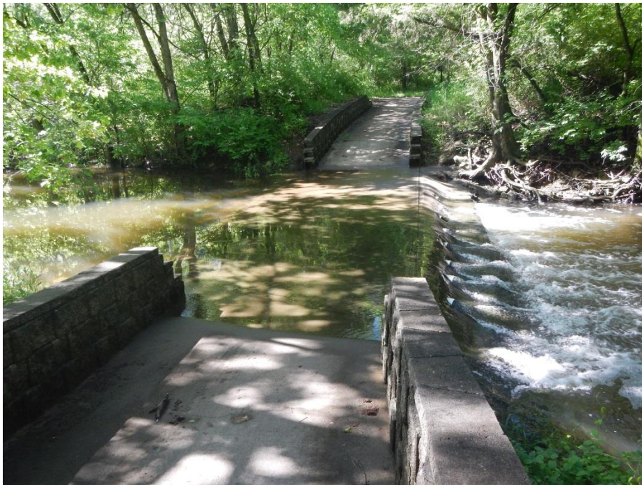
Photo 4. Site HFF downstream of Highway FF along Greenway Trail.
