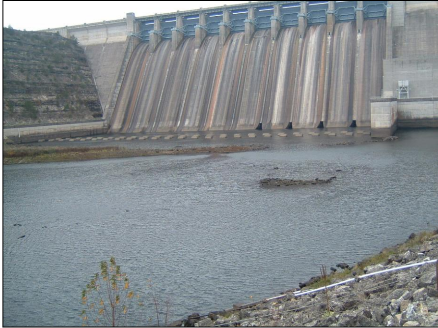
Figure 2.21: White River-below Table Rock Dam (7) (November 12, 2005)
