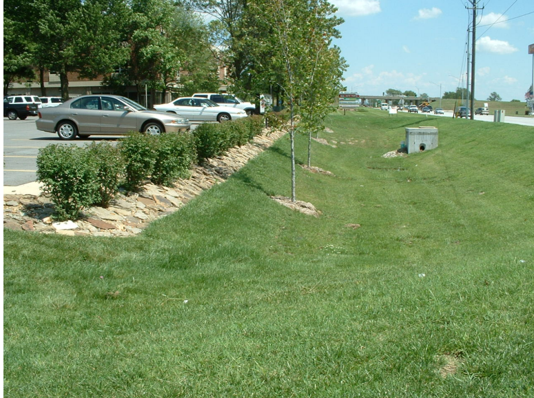
Figure 4. Extended detention basin for water quality treatment in Springfield. Vegetation slows and filters runoff from the parking lot. The concrete outlet structure is designed to slowly release the runoff over a 24-hour period, allowing sediment and associated pollutants to settle out.
