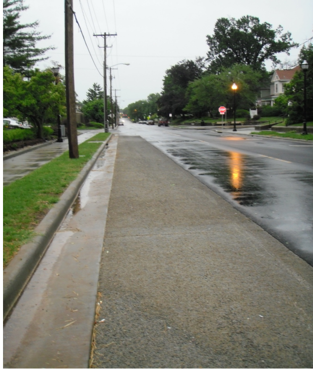
Figure 19. Pervious concrete on Walnut Street in Springfield.
