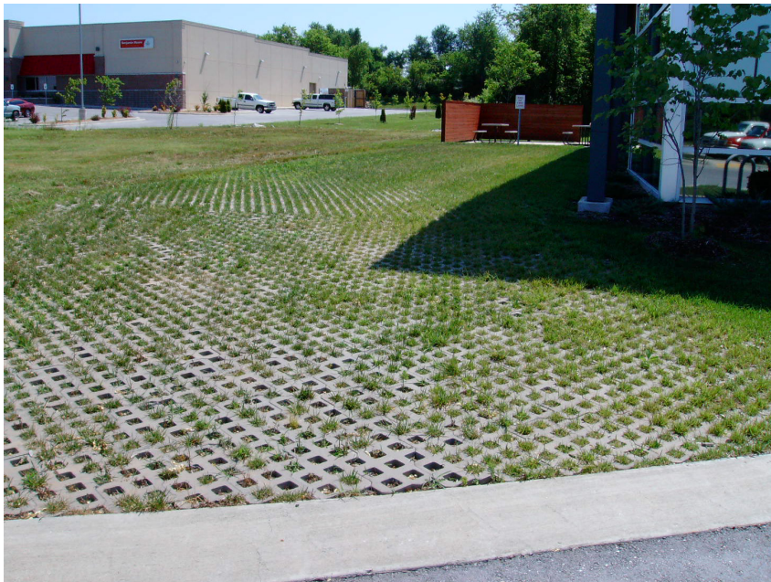
Figure 22. Grass pavers used for a building fire access lane in Springfield.
