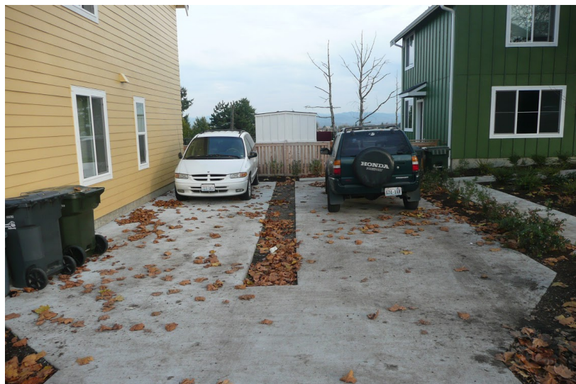
Figure 20. Shared driveway with pervious strip in the middle in Seattle, Washington (Arazan, 2008).
