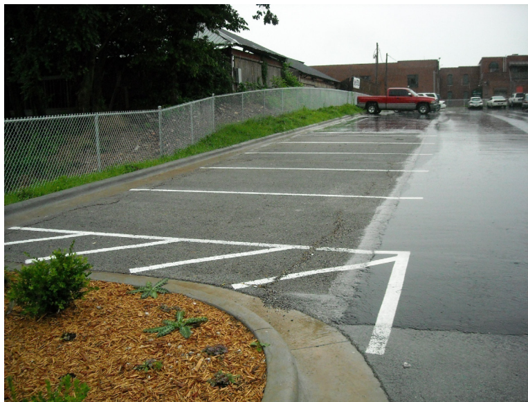
Figure 5. Pervious concrete (left) adjacent to regular concrete (right) on a public parking lot in Springfield. Pervious concrete allows rainfall to infiltrate, either into the underlying soil or into underlying gravel and perforated pipe, reducing the volume and/or velocity of runoff.
