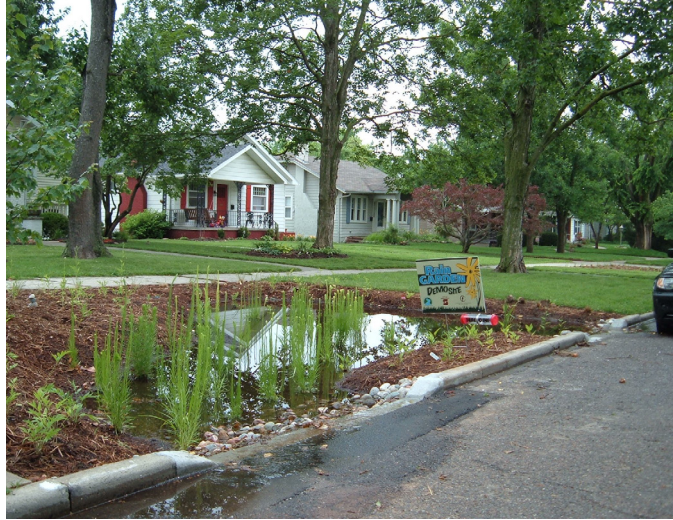
Figure 18. Street curb cut and rain garden on Weller Avenue in Springfield. The curb cut allows the street runoff to flow into the rain garden.
