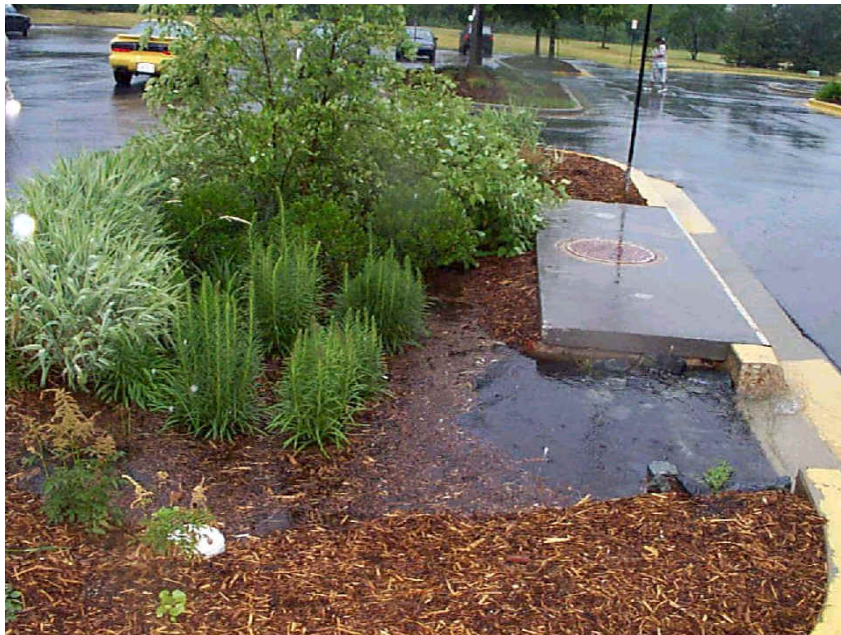
Figure 13. Bioretention in a parking lot island. This is an example of a small, distributed SCM used in LID design (University of Maryland, 2014).
