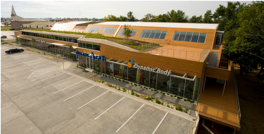
Figure 7. Green Circle Shopping Center, one of the first LID sites in Springfield (Green Circle Shopping Center, 2014). LID features include a pervious concrete lot, green roof, rainwater harvesting, shared parking, and tree preservation.
