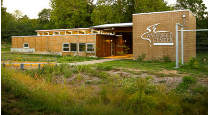
Figure 8. The C.W. Titus Education Facility at the Watershed Center in Springfield. It serves as a demonstration site for LID to educate the community about water quality protection (Watershed Committee of the Ozarks, 2014).
