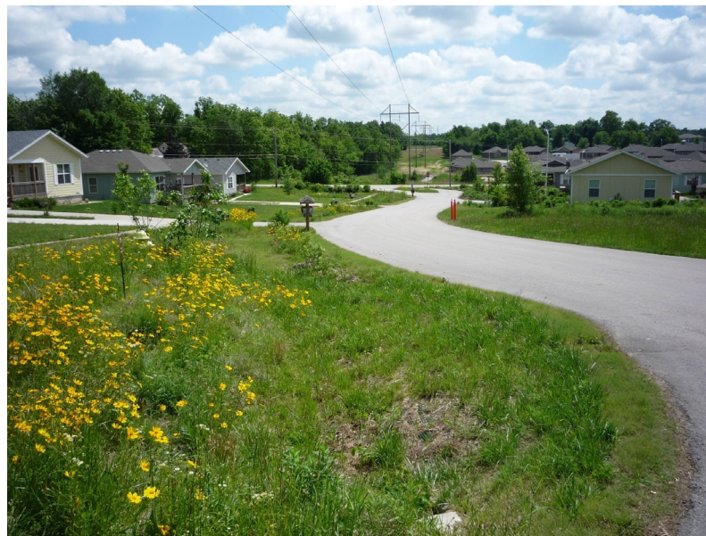
Figure 14. Legacy Trails LID subdivision developed by Habitat for Humanity in Greene County, Missouri. Site grading was minimized. Narrow, curbless streets and shared driveways minimize impervious cover. Roadside swales with native vegetation slow and filter runoff (Greene County Resource Management, personal communication, February 2014).
