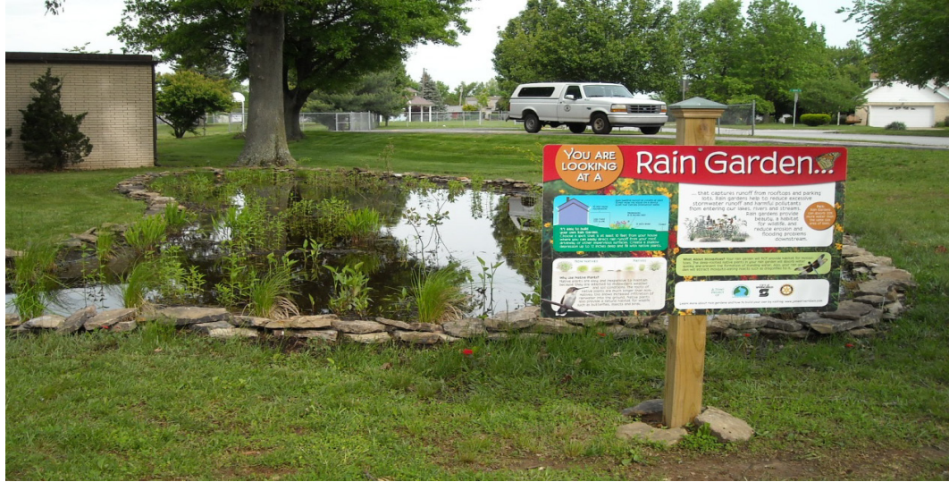
Figure 6. Rain garden at Horace Mann Elementary School in Springfield. Rain gardens are shallow planted depressions that reduce runoff through infiltration and evapotranspiration.
