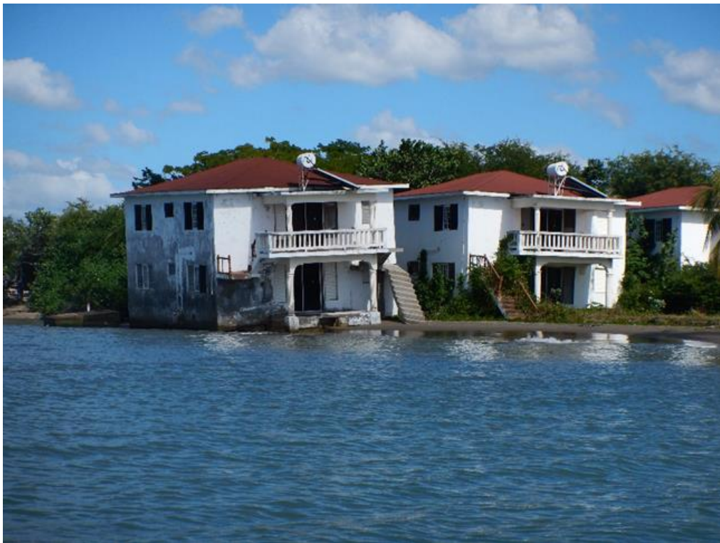
Figure 27. Property Damage Due to SLR and Shoreline Erosion. Picture taken in January, 2014.
