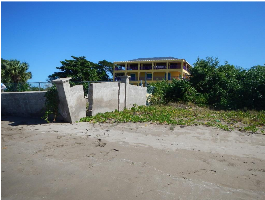
Damaged infrastructure (transect 440).
