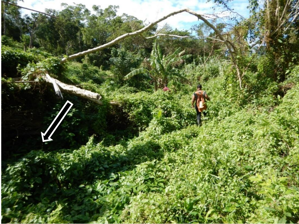
Appendix B-13. Point 10 – Sinkhole Because It Is Heavily Vegetated, Could Be a Deep Plunge Pool Migrating from the Head of the Incised Channel
