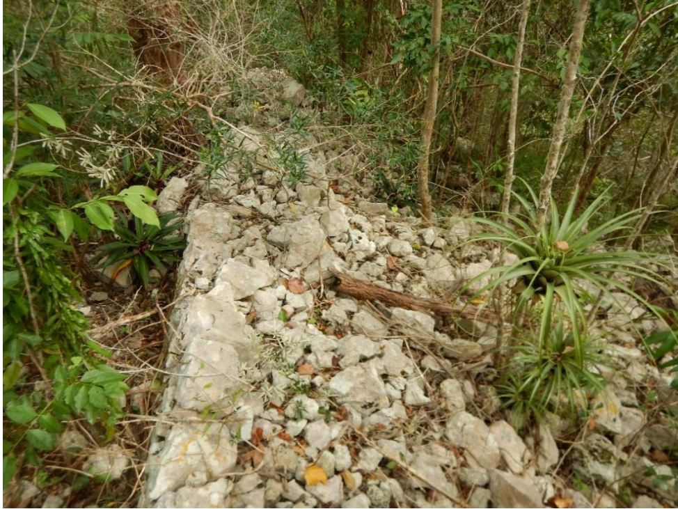
Appendix B-31. Point 26 – Boulder Wall, Although There Is No Evidence of Influence on Flow, It Indicates the Deposition of a Large Amount of Large Sediment Here
