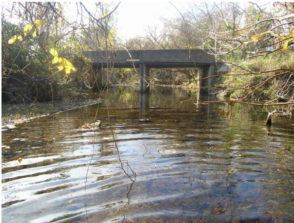
Site JC3 (Main stem Jordan Creek at Fort Avenue): Downstream view showing base flow (Staff gage is located on bridge base at right of picture).
