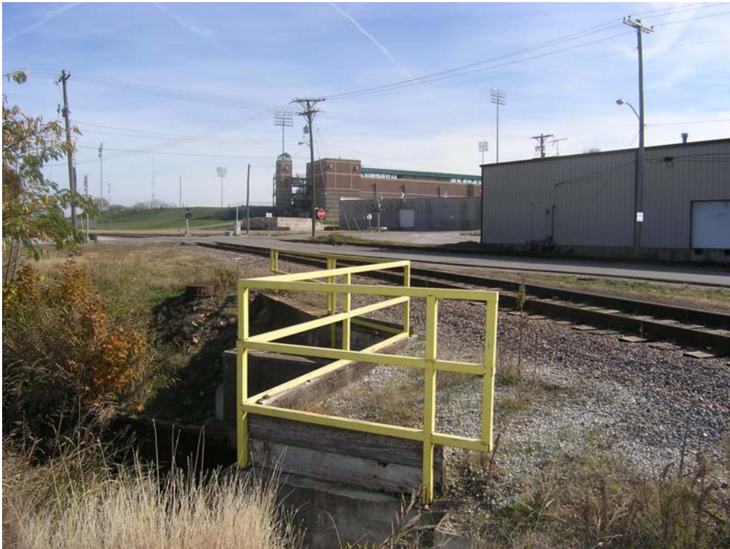
Upstream view of baseball stadium from site SB2.
