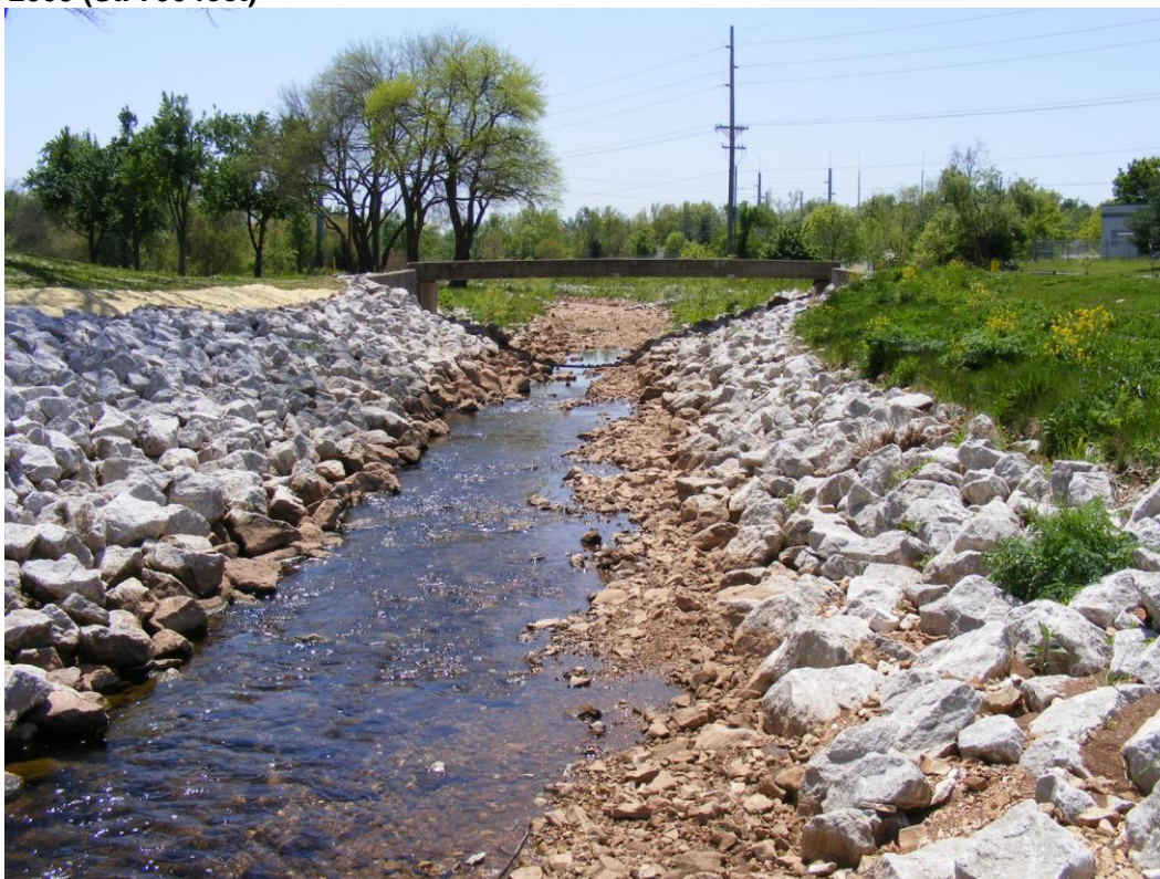
Picture 16. AFTER - Bank angle lower and toe rock above second cart bridge looking downstream May 2008 (St. 800 feet)
