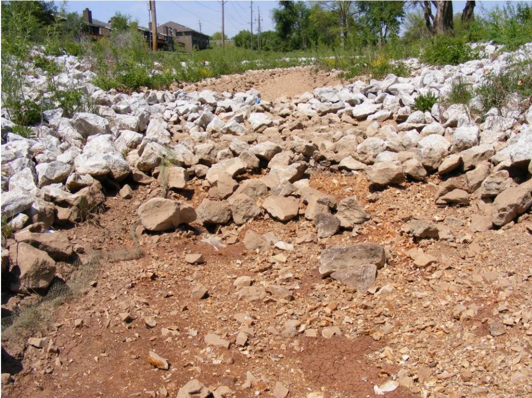
Picture 7. Lower grade control structures near the end of Golf Course Reach looking upstream May 2008 (St. 1,150 feet)
