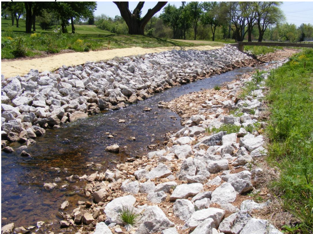
Picture 4. Upstream of lower cart bridge looking downstream May 2008 (St. 600 feet)
