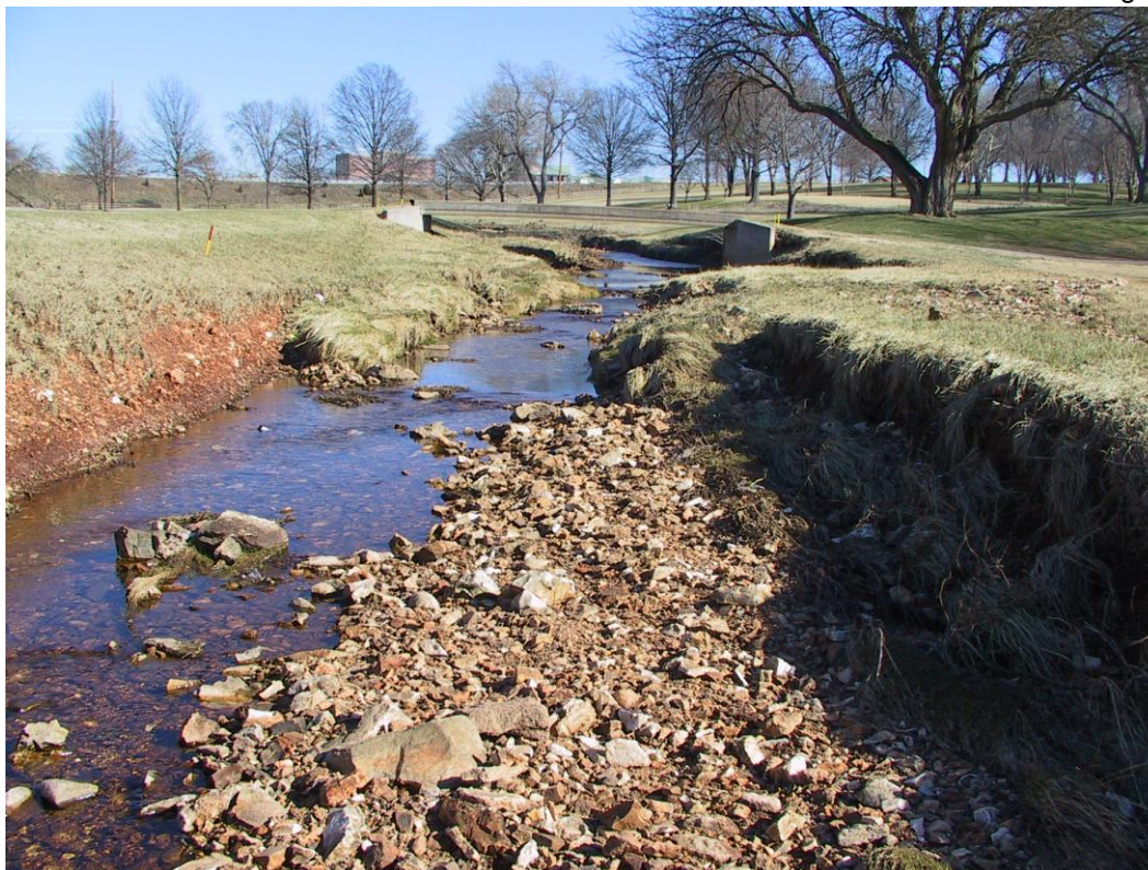
Picture 13. BEFORE - Riffle crest, bank failure, poor riparian conditions below second cart bridge looking upstream December 2004 (St. 850 feet)
