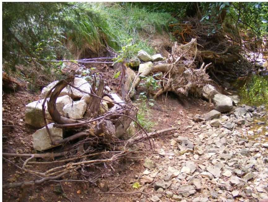
Picture 26. Possible bed elevation lowering at root wad structures, July 2008 (St. 1,320 ft)
