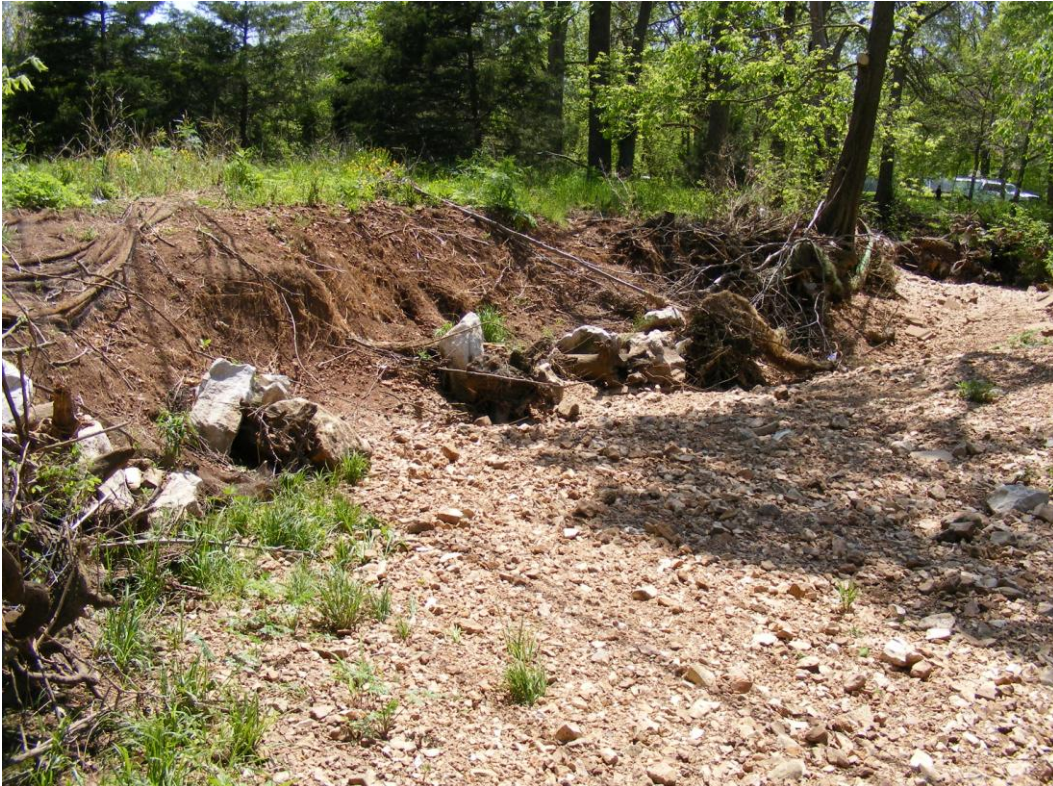
Picture 9. Root wads at meandering sub-reach looking downstream May 2008 (St. 1,650 feet)
