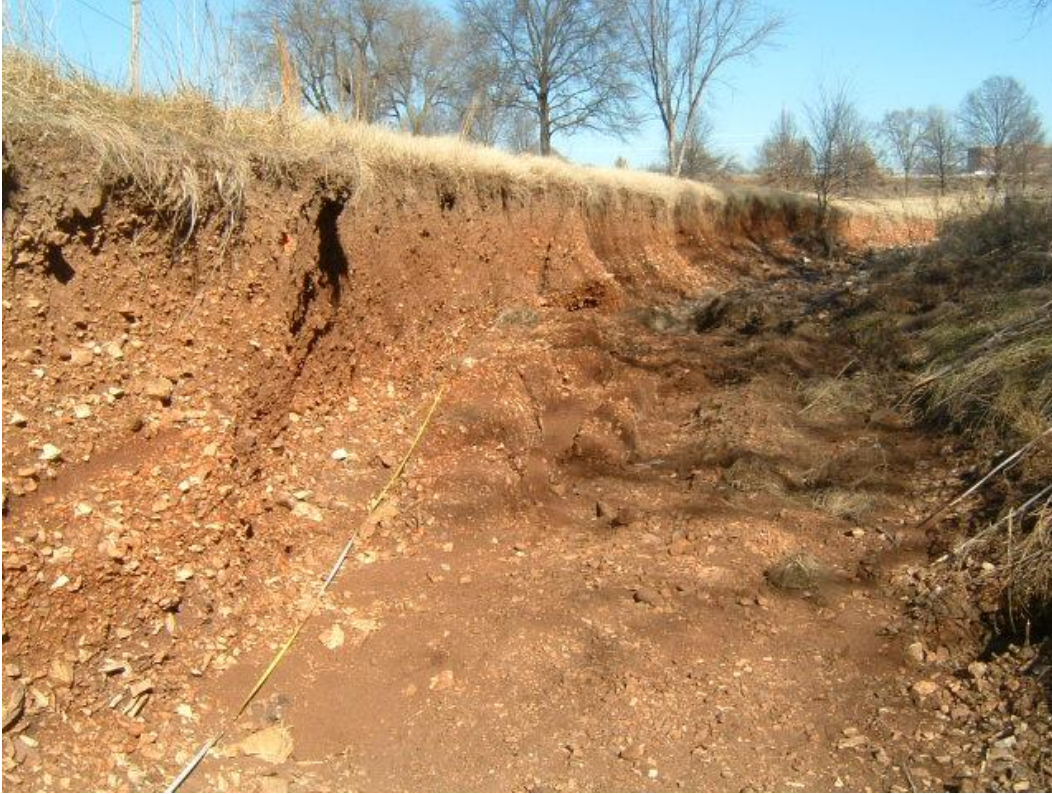
Picture 17. BEFORE - High west bank failure looking upstream January 2006 (St. 1,050 feet)
