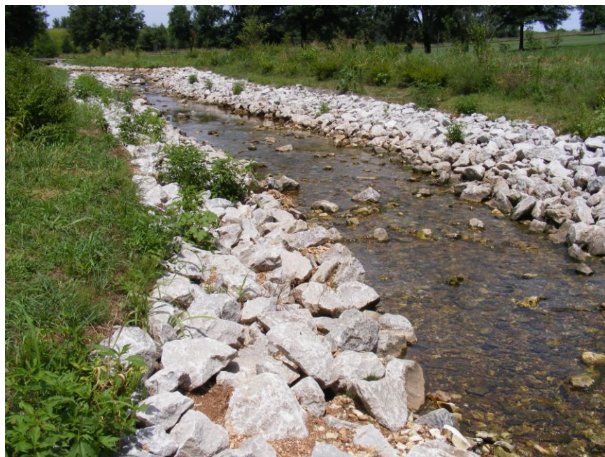
Picture 22. Step-pool reach below first grade control structure, July 2008 (St. 500 ft)
