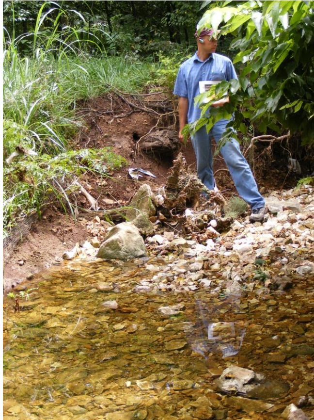
Picture 27. Aggrading bed at root wad structures, July 2008 (St. 1,500 ft)
