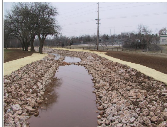
Looking downstream from lower cart bridge to station 1,000
