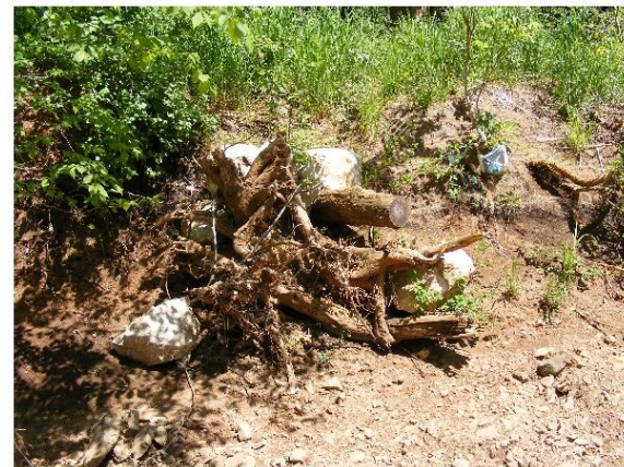
Example of root wad installed at station 1,580 feet
