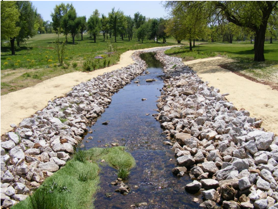
Picture 2. Downstream of upper cart bridge looking downstream May 2008 (St. 120 feet)
