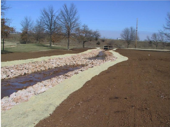
Above station 500 feet looking upstream
