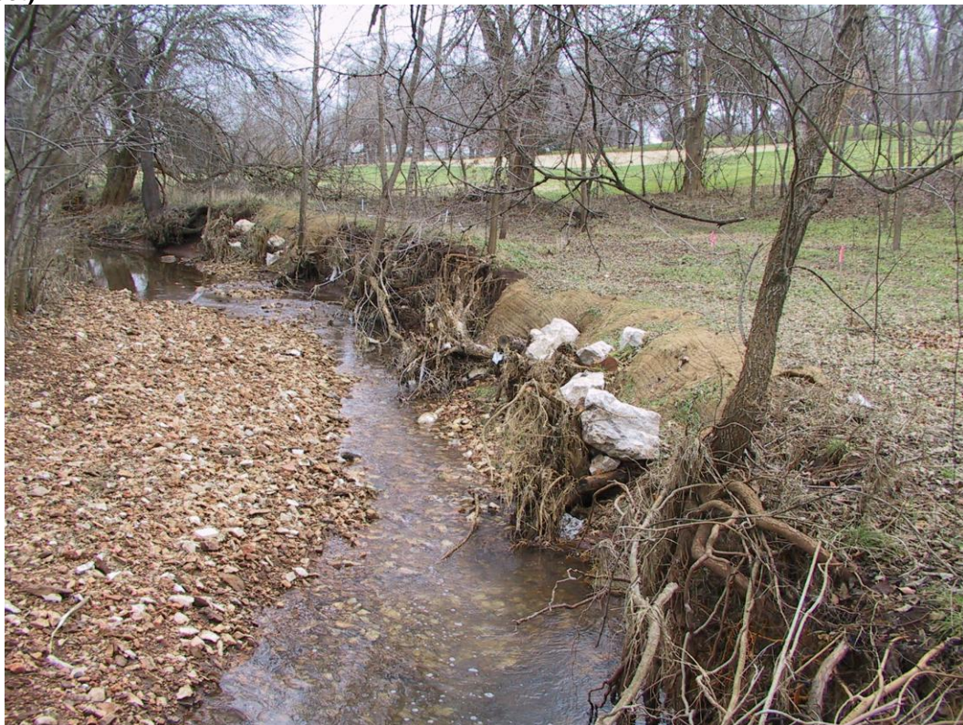
Picture 20. AFTER - Root wads installed along meandering reach looking upstream March 2007 (St. 1,500 feet)
