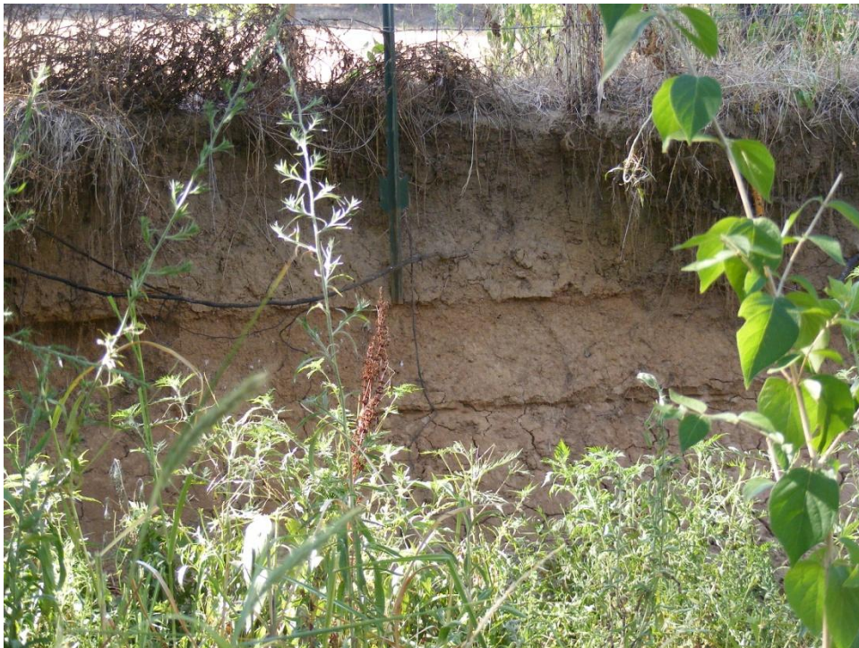
Photo 4. Knickpoint Reach (3,600 ft) left bank erosion.
