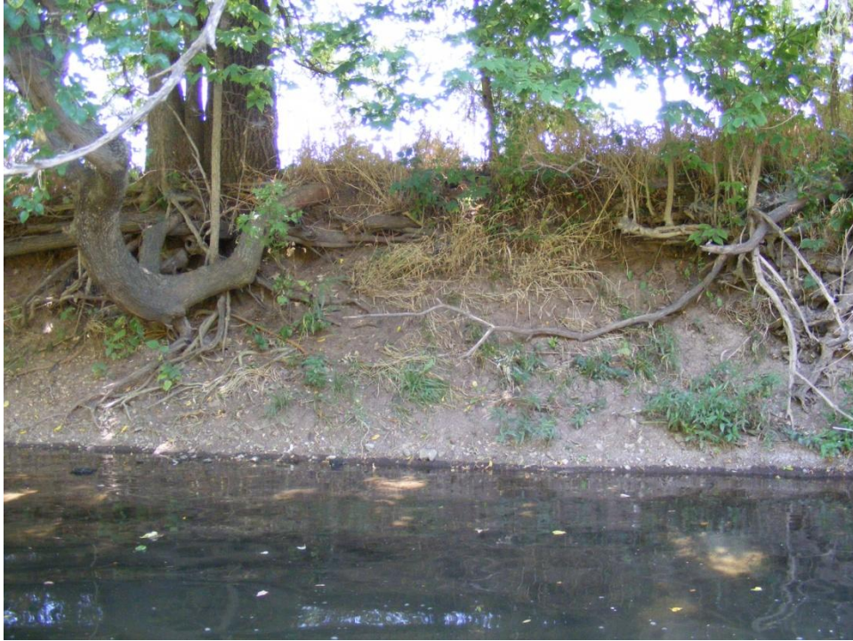
Photo 27. Gravel Bed Reach (500 ft) looking at the right bank.
