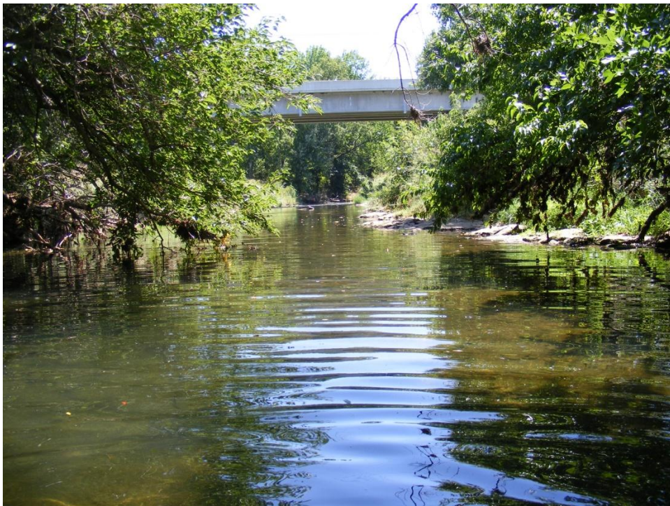
Photo 28. Bedrock Bed/Bridge Reach (250 ft) looking downstream toward Republic Road Bridge.
