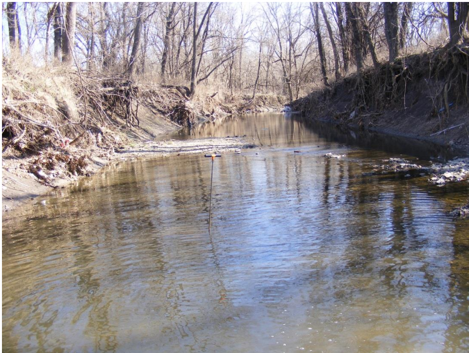
Photo 10. Example of main channel widening - high vertical banks, exposed tree roots, and slumping are indicators of erosion.
