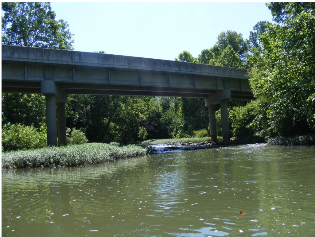
Photo 4. Cox Road Bridge at station 2.7 km
