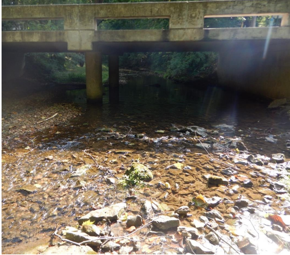
Photo 3. Looking upstream at the FR 144 (Catalpa) Bridge. PC_Cat (8-7-18)
