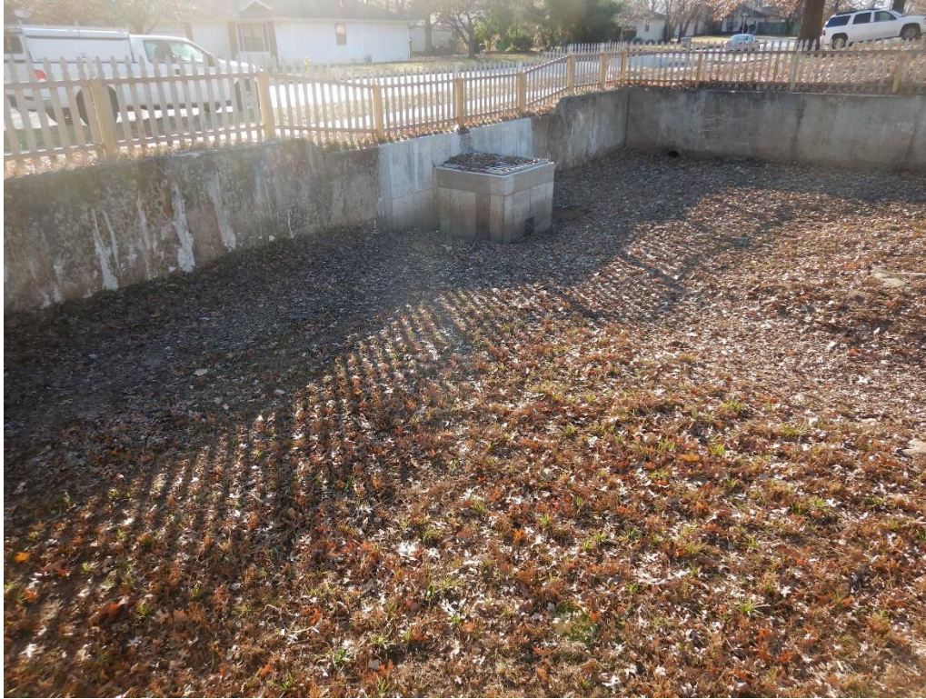
Photo 5. New outlet structure at the Seminole detention basin (Dec. 3, 2019).
