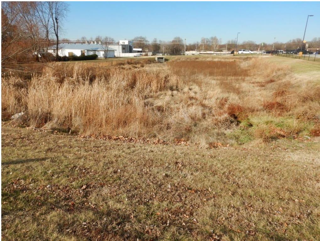
Photo 6. Wetland plants were added to the Frisco Trails detention basin (Dec. 3, 2019).
