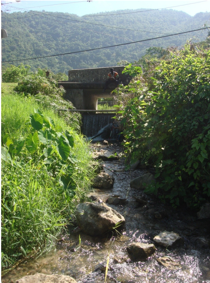
River Top Bridge- Upstream (River meter 1077)
