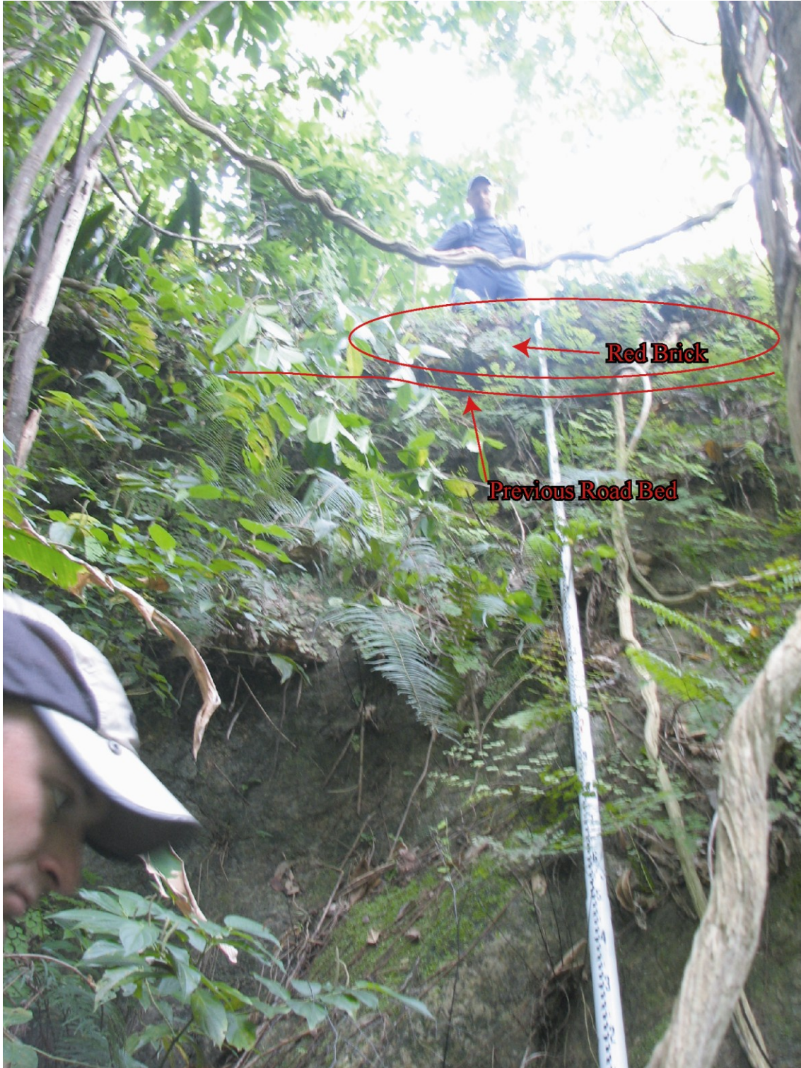
Figure 28. Old Great House Road bridge elevation. Notes: Previous road elevation of the bridge is about four meters above the present channel thalweg. Oral history accounts indicate that the bridge structure was about one meter above the bed at river meter 607.
