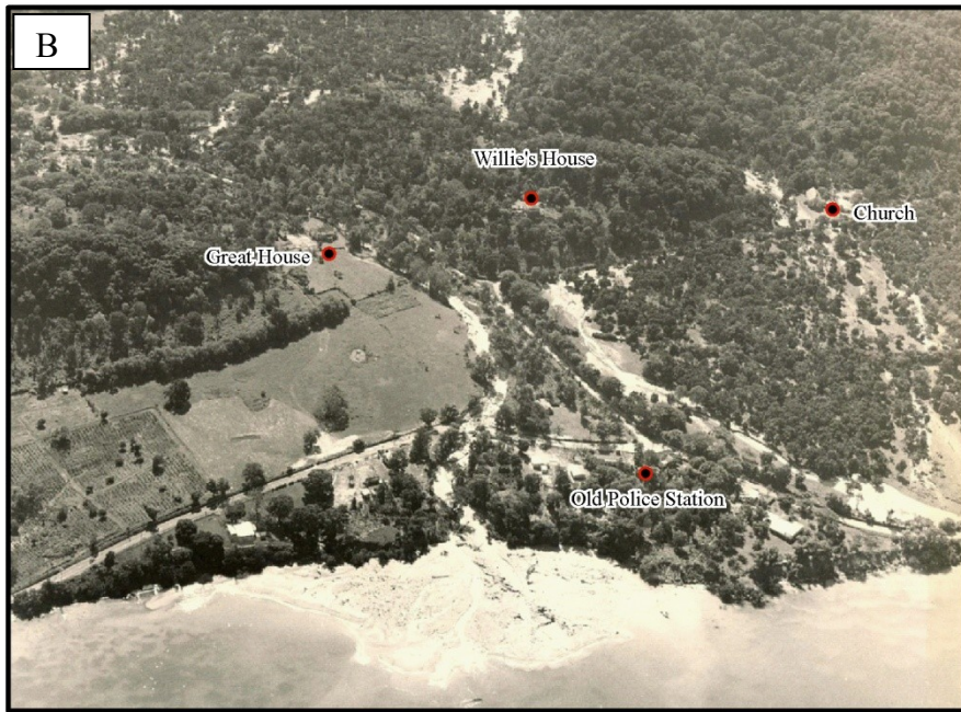
Figure 30. Debris Fan Formation. Aerial photography from 1968 (A) illustrates how the debris fan was much smaller than the debris fan post 1979 (B).
