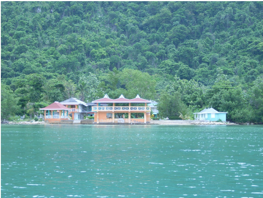
Appendix A- 23. RIMG0146 – Riprap and Sea Wall.
