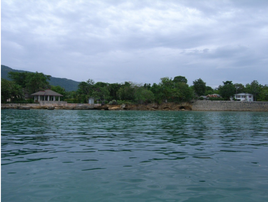
Appendix A- 4. RIMG0016 - Sea Wall and Bedrock.
