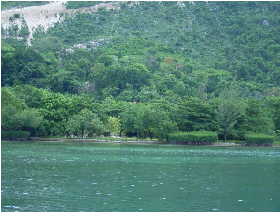
Appendix A- 25. RIMG0152 - Riprap and cultured vegetation below new development.
