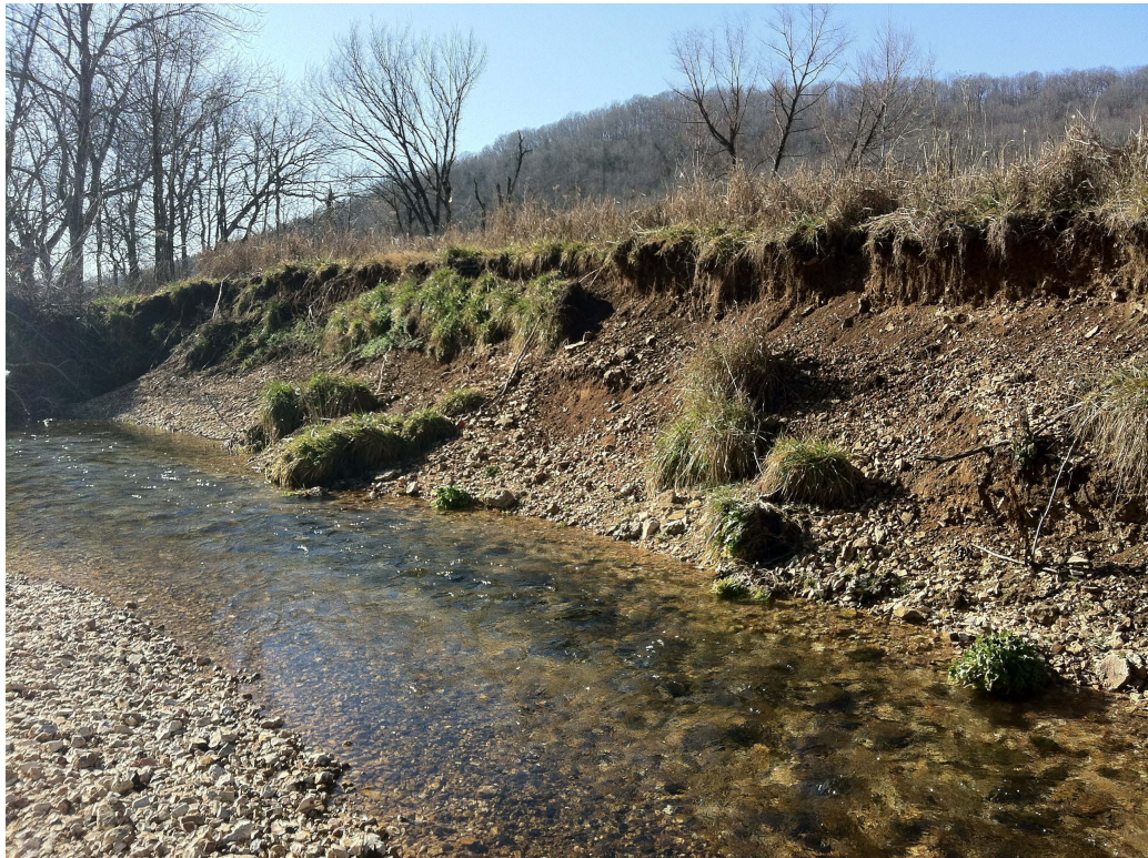
Adjacent of megabar at FS11-12 with erosion into floodplain coluvium
