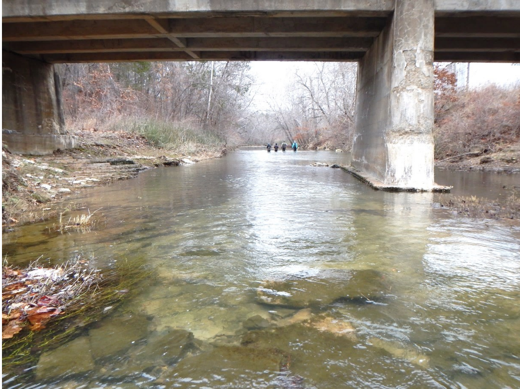
Straight bedrock reach under St. Joe Parkway at R-km 3.57.
