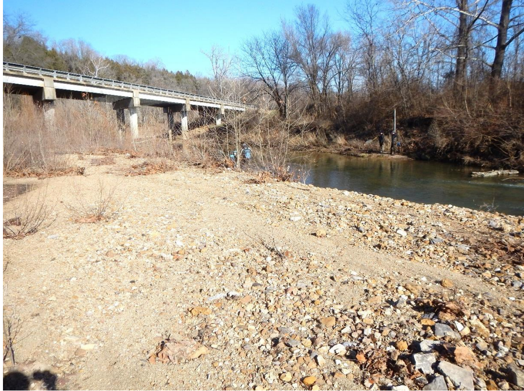
Active bar deposit above Cedar Falls Road at R-km 1.25.
