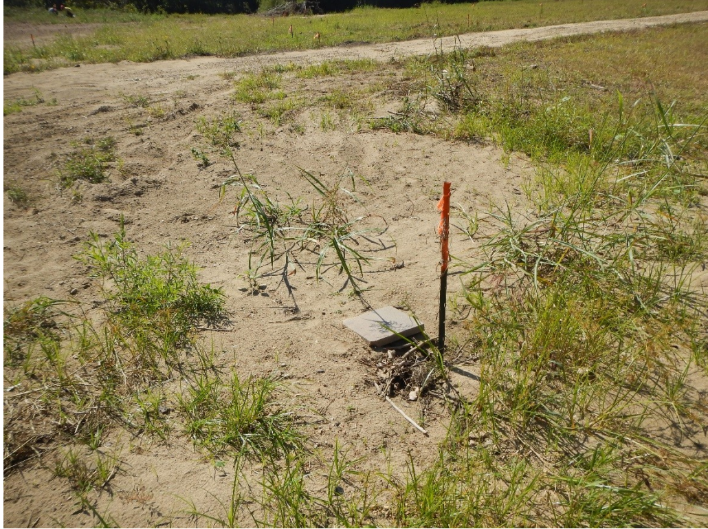
Sampling block 25 with erosion around block (9/17/15).
