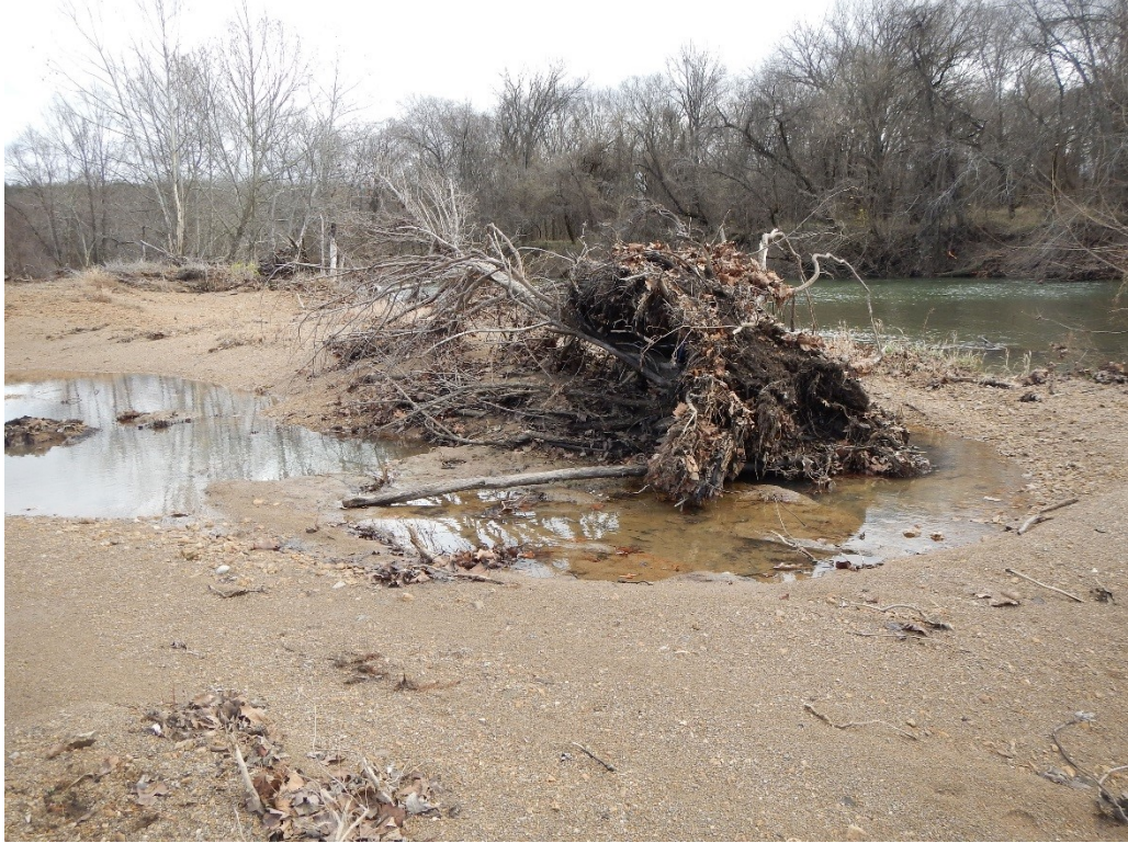
Erosion of inlet around large woody debris (12/14/15).
