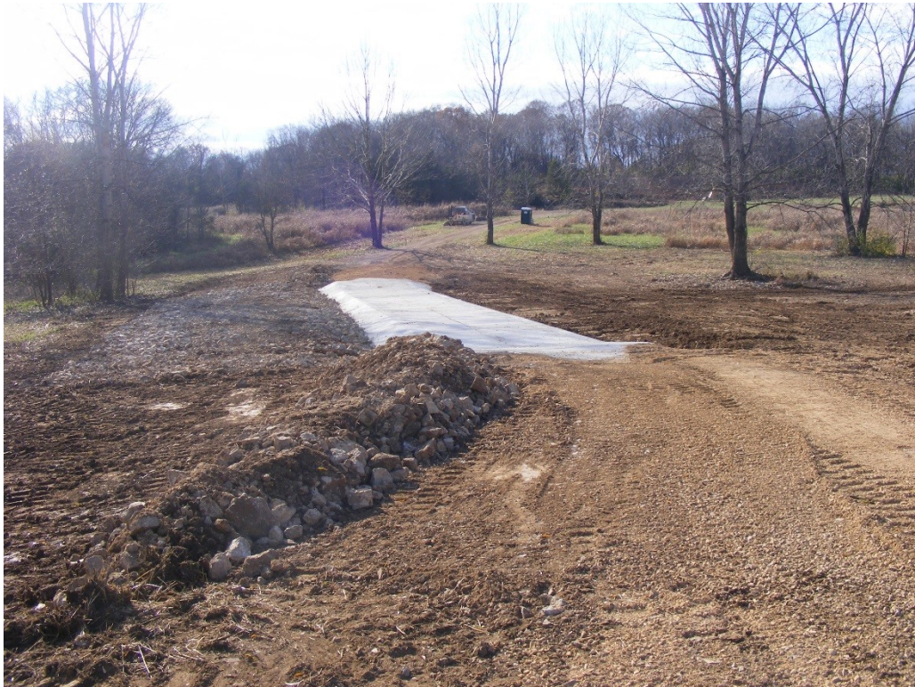
Concrete spillway (11/21/16).
