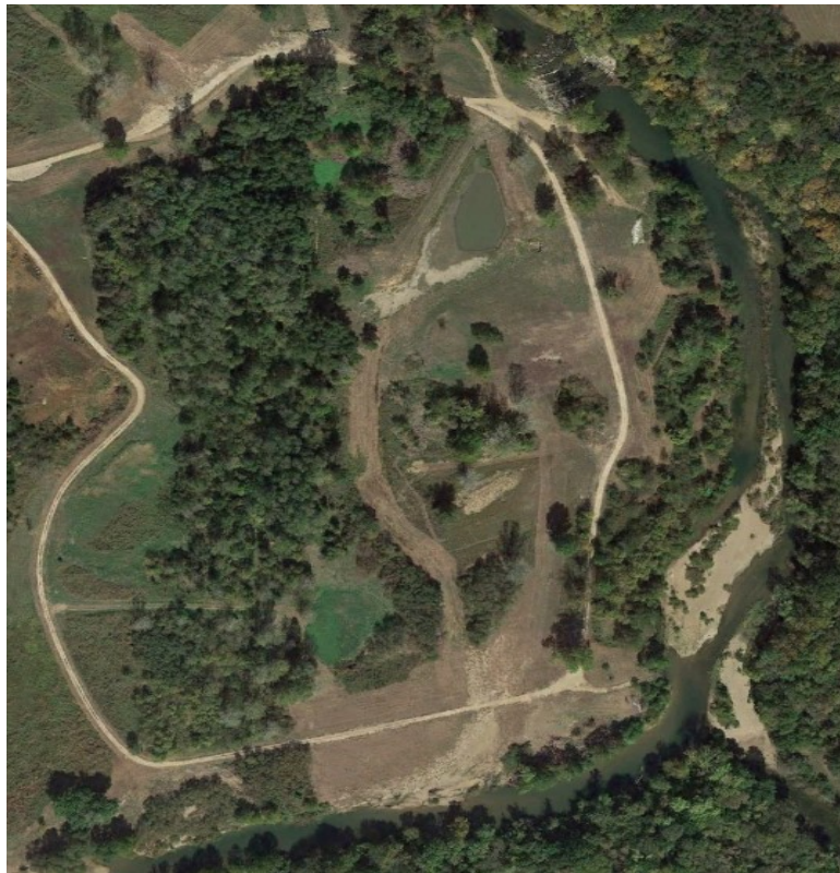
Figure 15. BRLRS site pre-construction (November 2013) (top) and post-construction (October 2015) (bottom) (Google Earth Pro, 2016).
