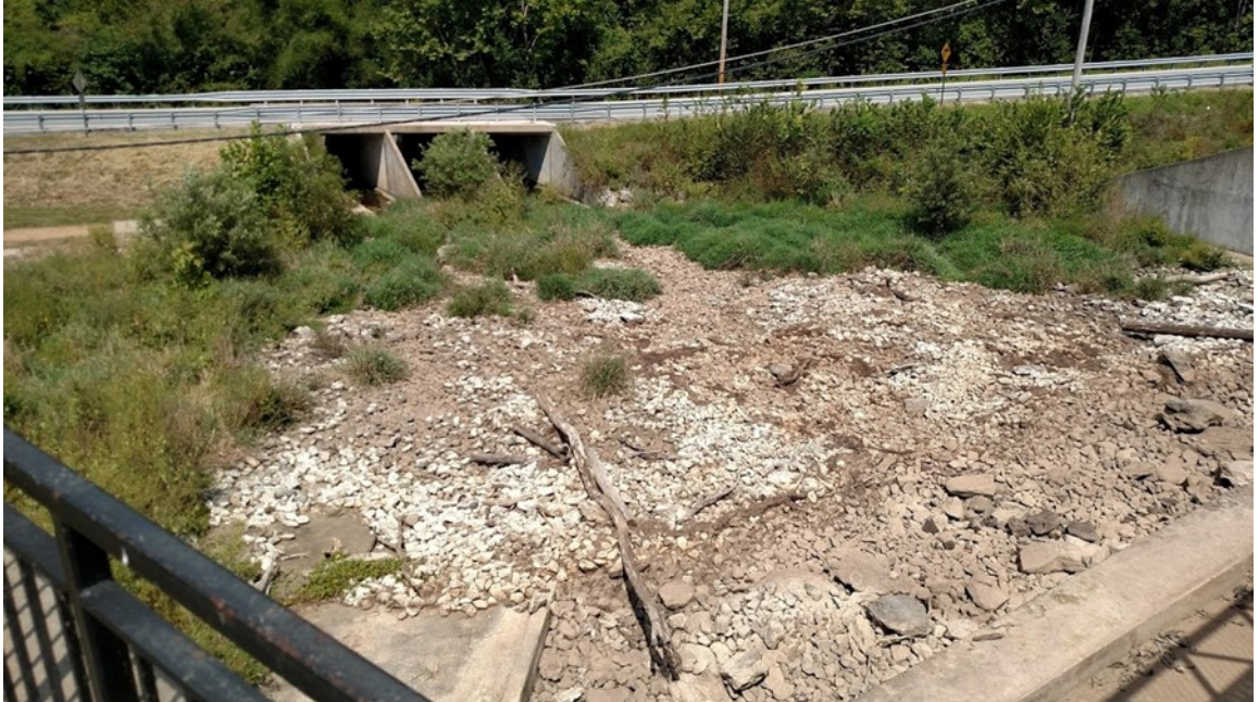
Figure 11. Valley Water Mill Reservoir spillway and culvert
