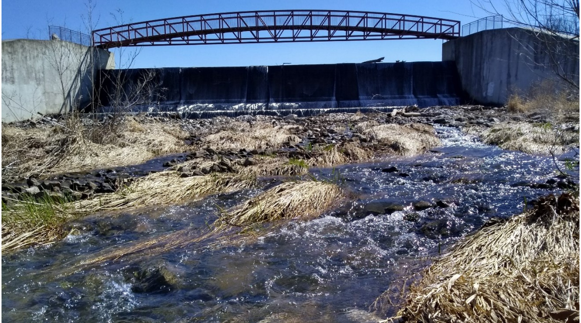
Figure 10. Valley Water Mill Reservoir dam overflow
