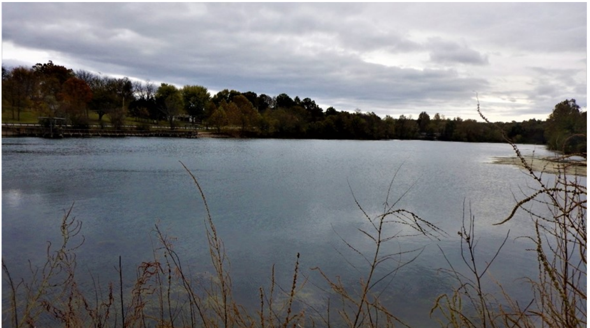
Figure 9. Valley Water Mill Reservoir
