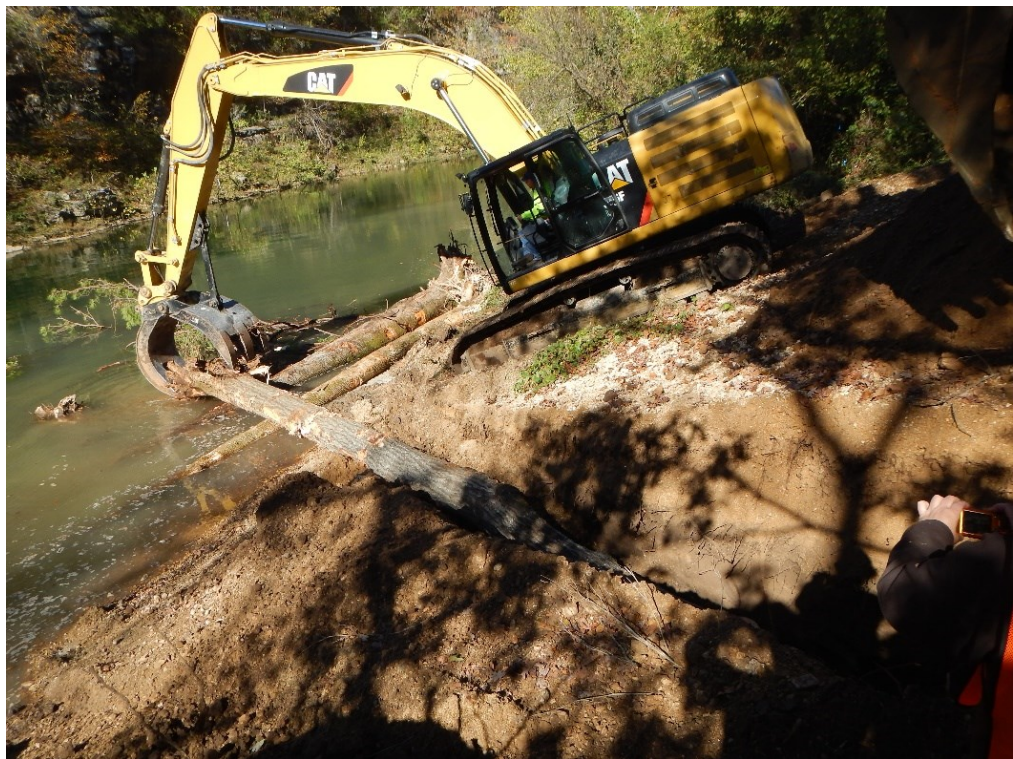
Figure 6. Excavator placing logs in a trench perpendicular to flow positioned over key pieces.
