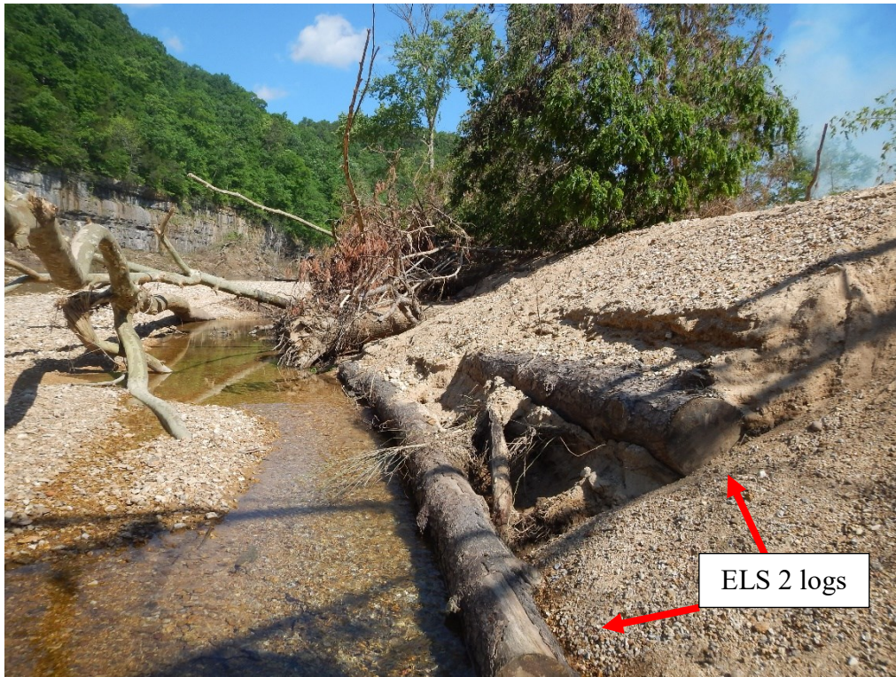
Figure 43. Deposition caused by April Flood at ELS 2 where bank angle lowered. Arrows show cut ends of logs in ELS 2.
