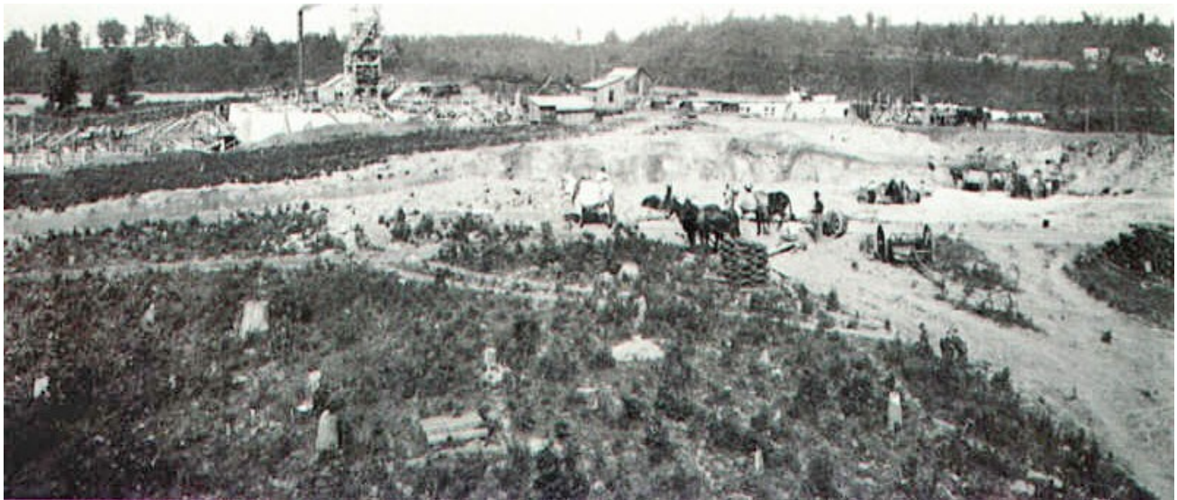
Figure 8: Bonne Terre surface mining operations, 1866. Mining from shallow pits and surface deposits was the primary method of ore harvesting until 1869. Image source: www.rootsweb.com
