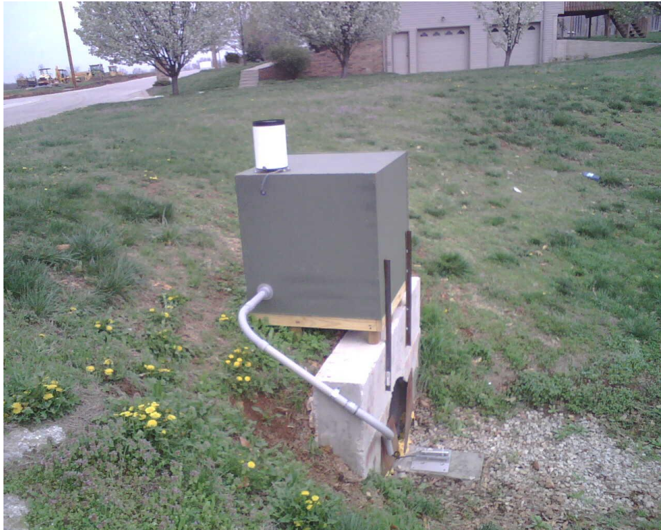
Figure 3. Monitoring Station Installation
