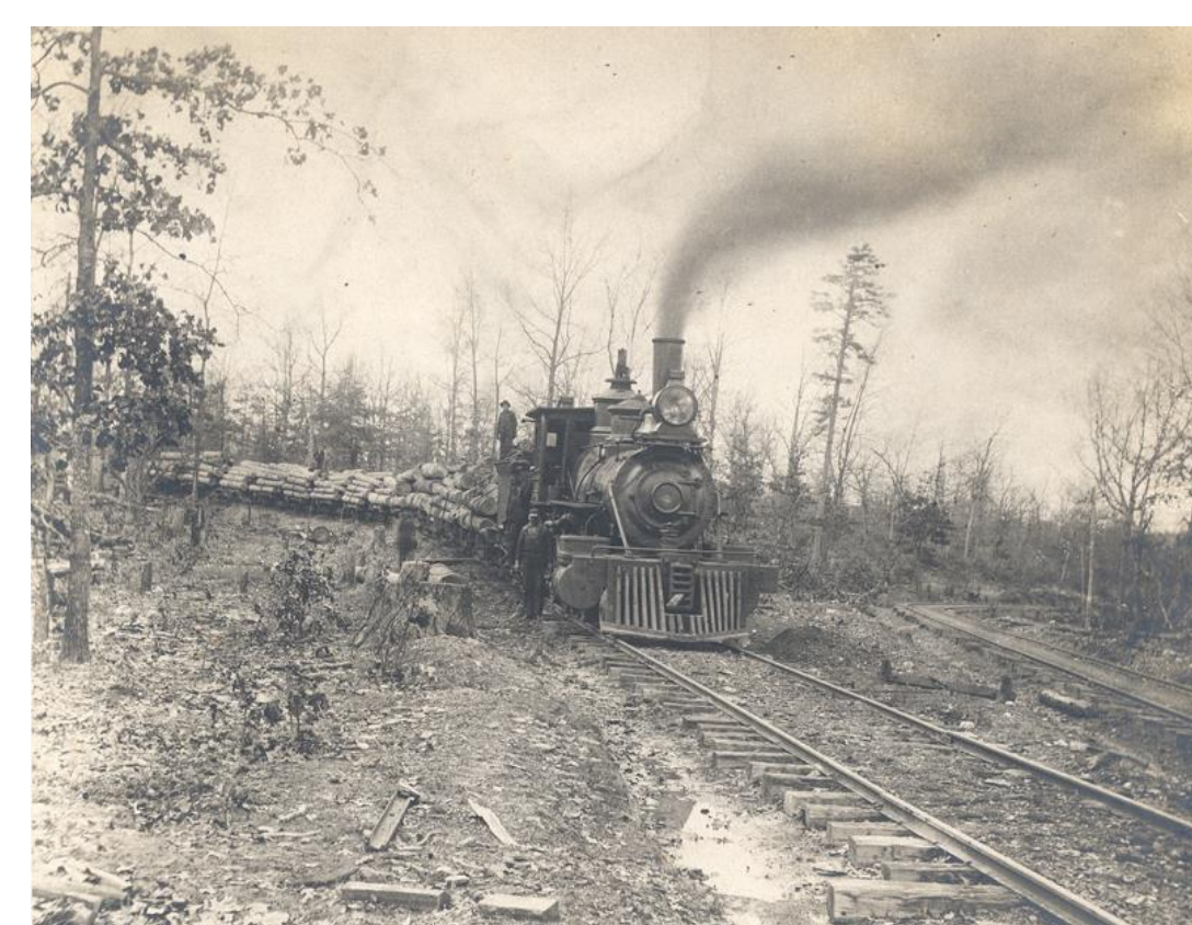
Photo 6. (above) Tram railways were used to move saw logs across the Current River to the mill at Grandin. (from Western Historical Manuscripts Collection—University of Missouri)
