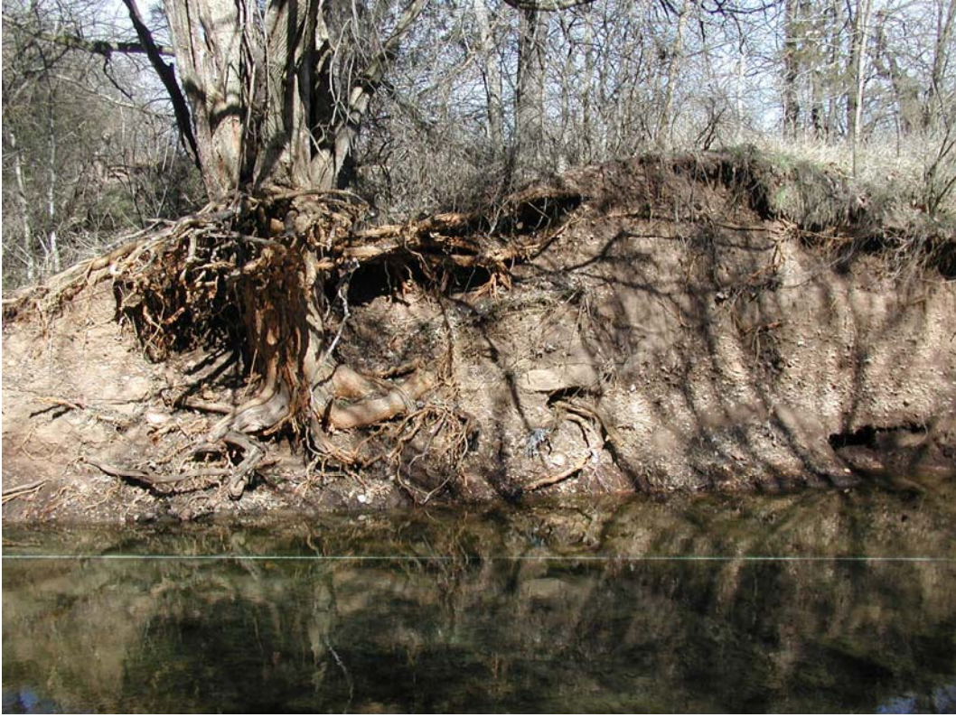
Picture 25. Disturbance reach cutbank (800 m)
