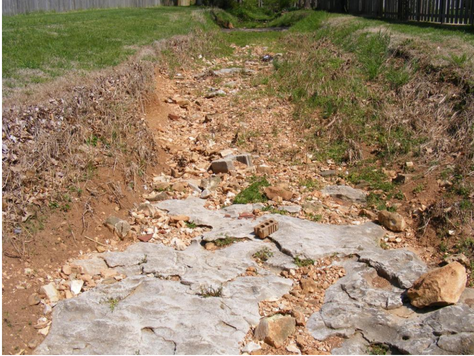
Picture 27 - Grass channel bed-upstream (4-29-08)
