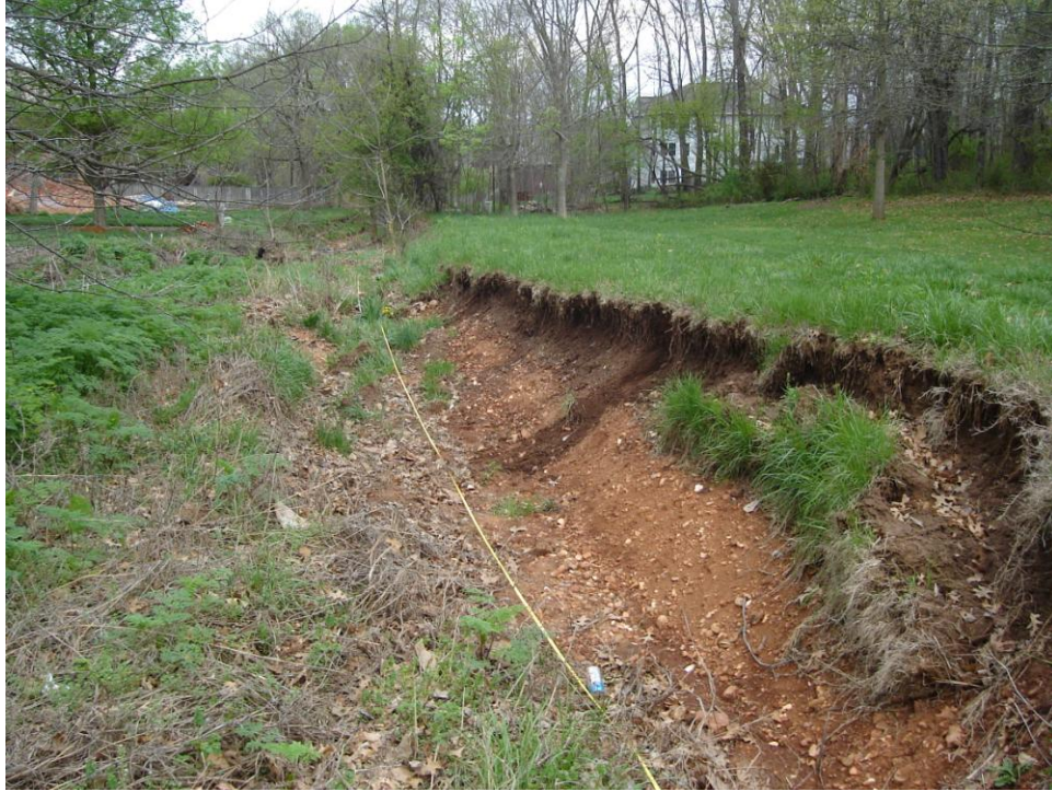
Picture 13 – Lower on of “double thalweg” at 100ft (sub-reach #4b)
