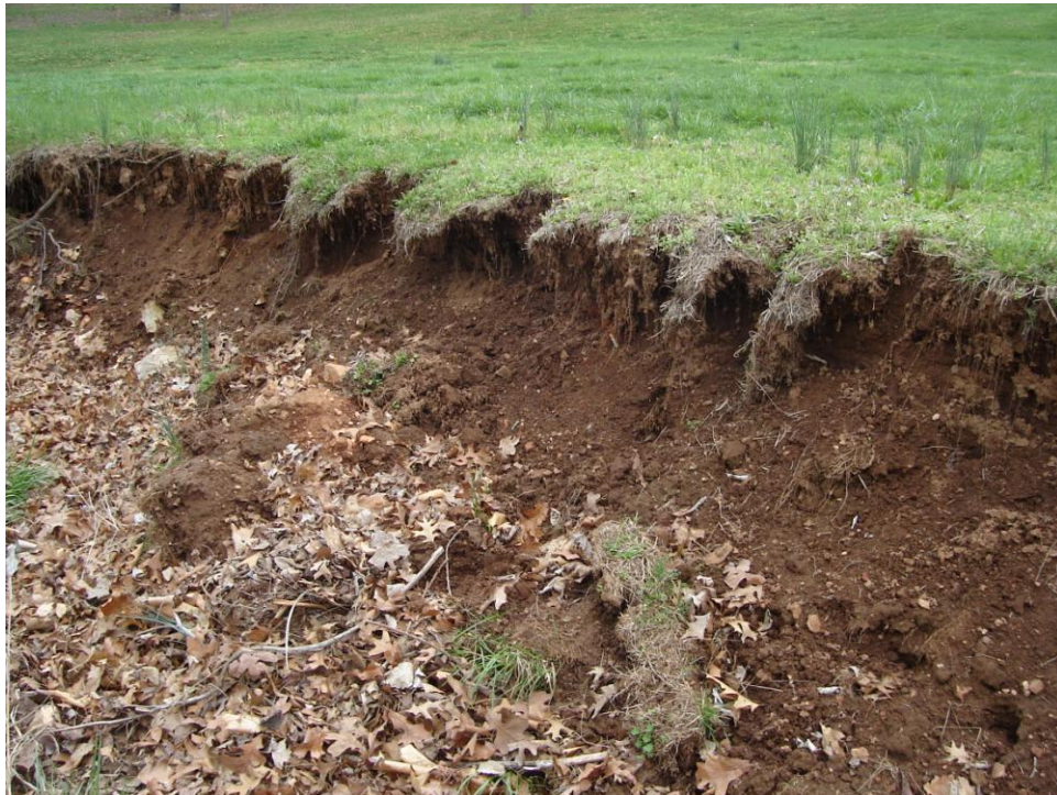
Picture 8 – Eroding bank at 400ft (sub-reach #3)
