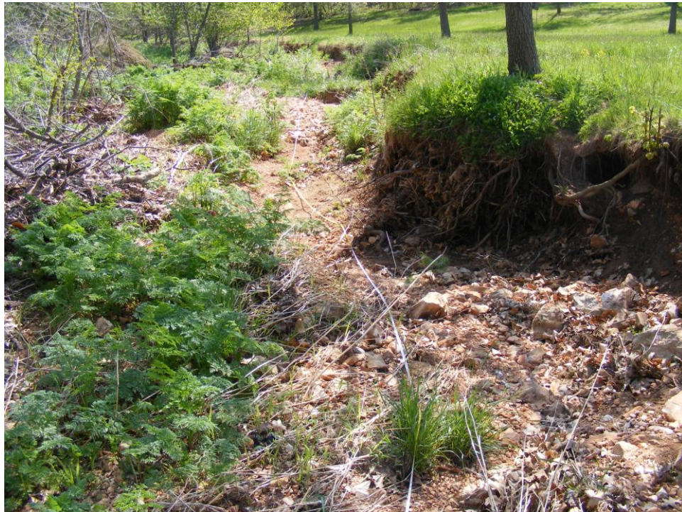
Picture 24 - Scour pool around a tree root at 310 to 340 ft (4-29-08)
