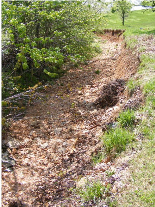
Picture 32 – Lower portion of sub-reach #2 (4-29-08)
