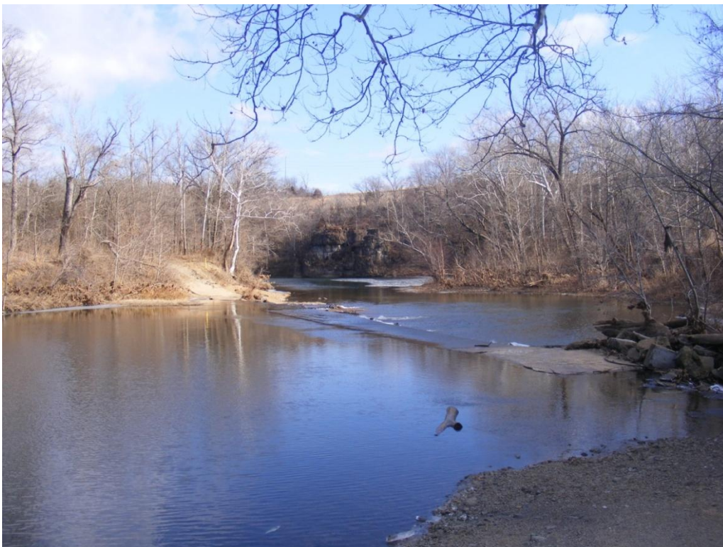
Looking downstream toward low-water bridge
