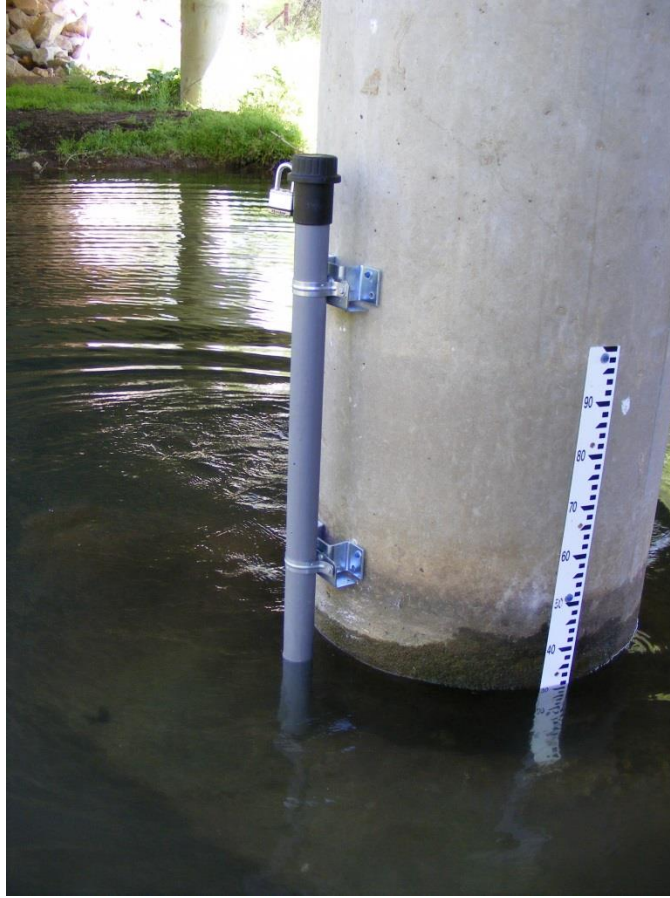
Photo 7. Levelogger installation at site AC03.
