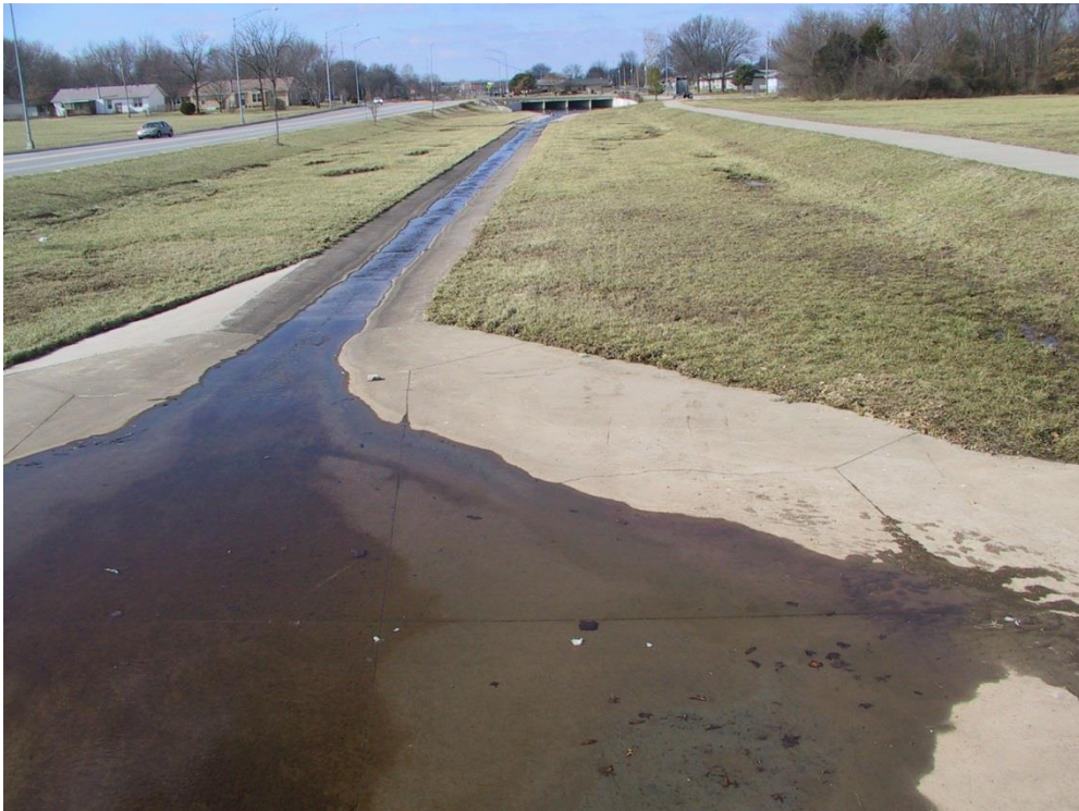
Photo 4. Concrete low flow channel and mowed turf grass riparian corridor downstream of Campbell Avenue.
