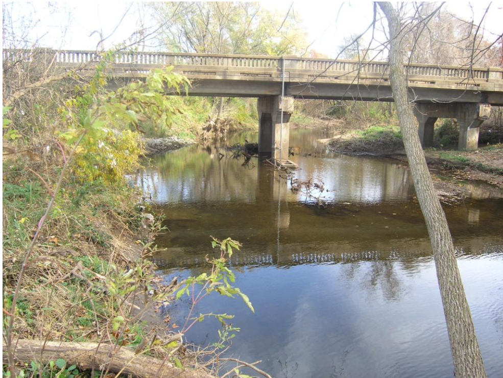
Site WC1 (Wilson Creek at Scenic Avenue): Upstream view showing baseflow. USGS gage is obscured by foliage at right of photo, gage sensor pipe on central bridge pier
