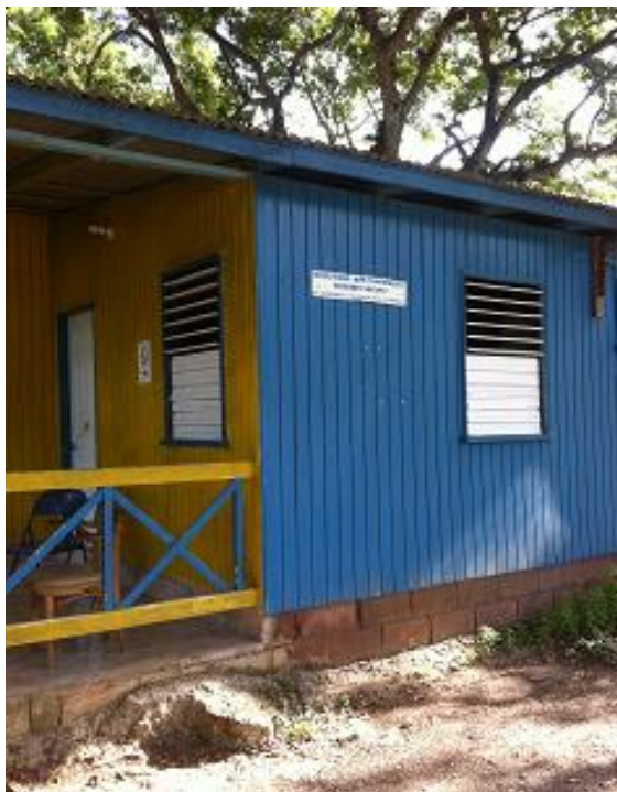
Figure 25. BBFFS Office, image taken January 2014.
