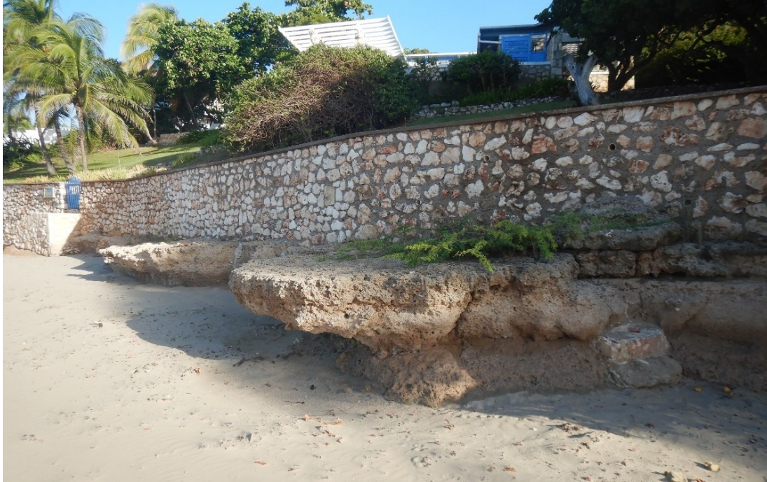
Figure 23. An example of an eroding beach in front of a stone wall at Calabash Bay (03/18/2021).
