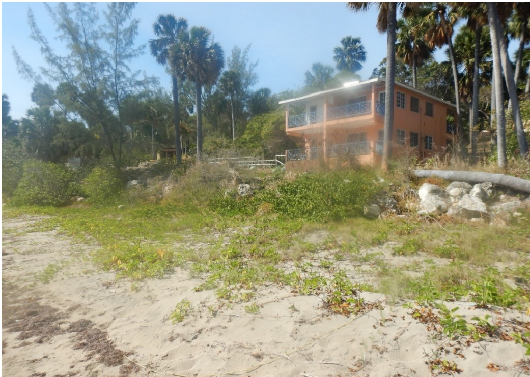
Rip-rap on the backbeach at a beach house at Billy's Bay.
