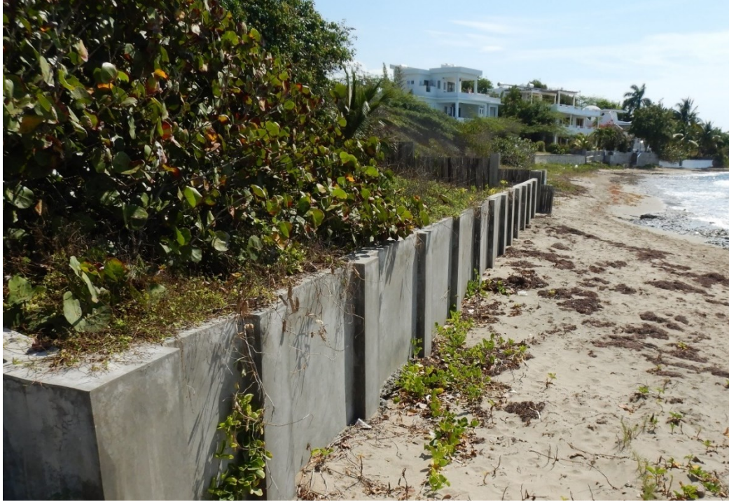
A narrow beach with a concrete wall on the backbeach, preventing beach propagation at Calabash Bay.
