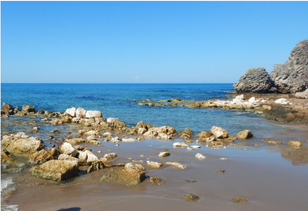
Two groins built with rocks at Mahoe Bay.
