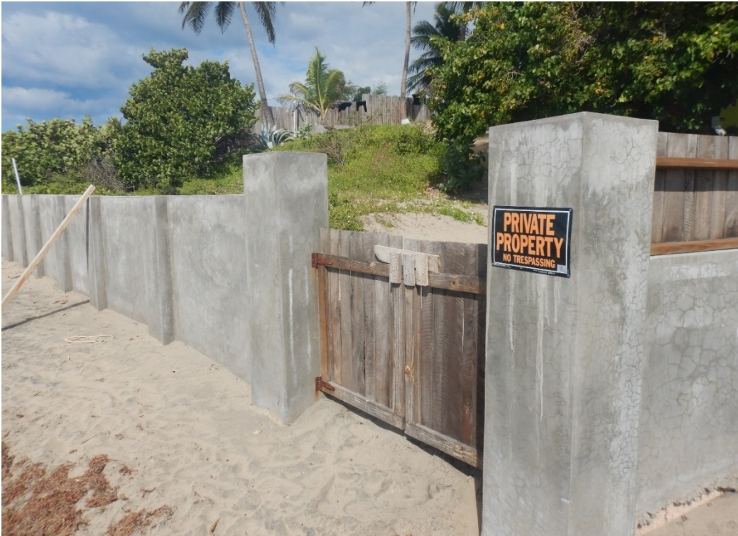
Cement wall built on the back beach at Old Wharf.
