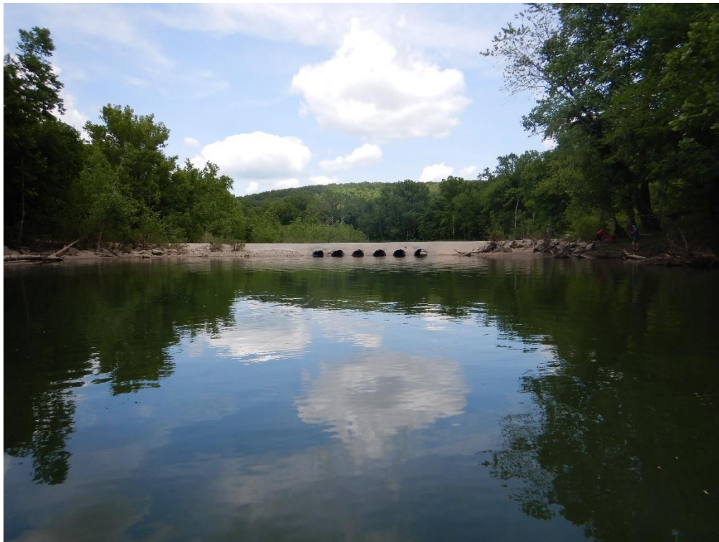
Photo 6. Low-water bridge downstream of RC8 (5/31/2019).
