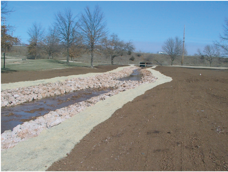
Above station 500 feet looking upstream
