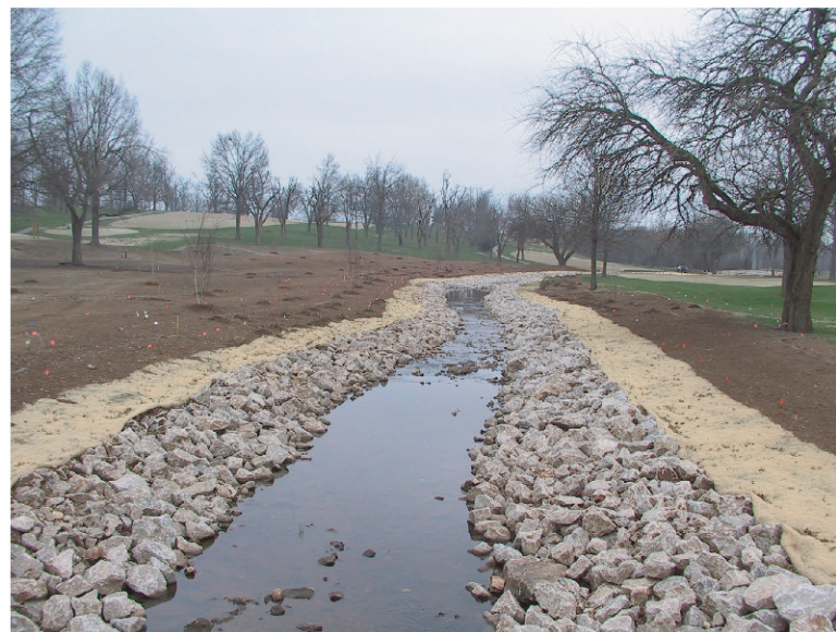
Looking downstream from station 100 feet at cart bridge
